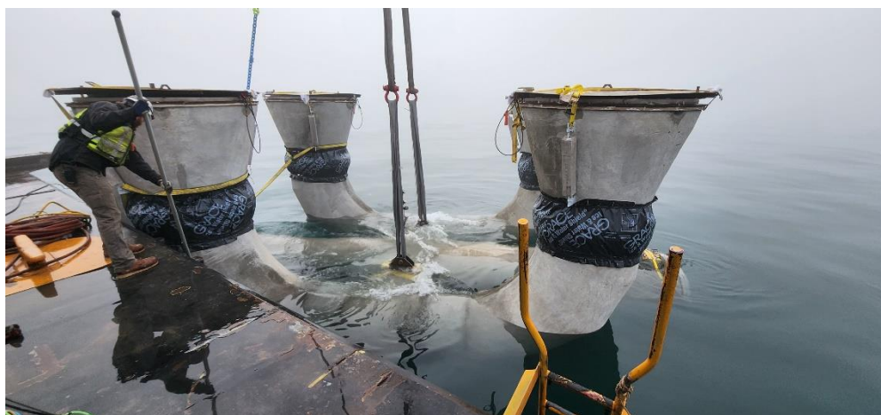
Intake structure submerged into position.
