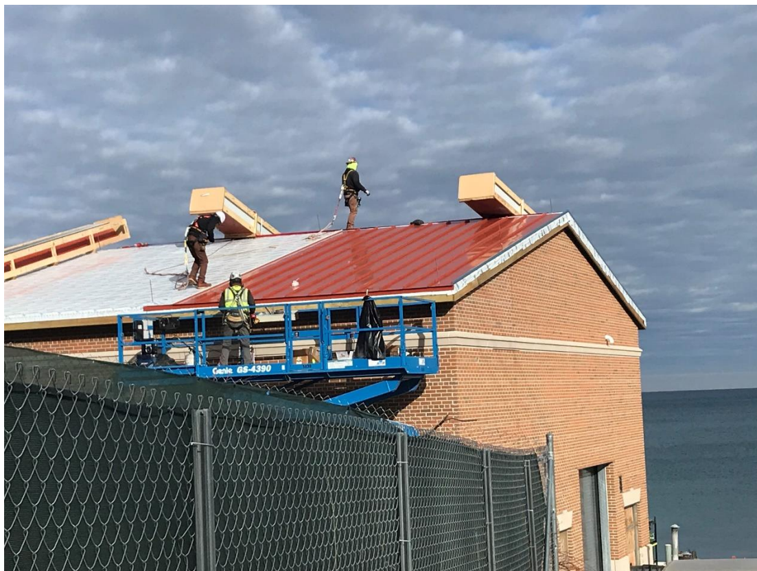
Standing seam metal roof installation activities.
