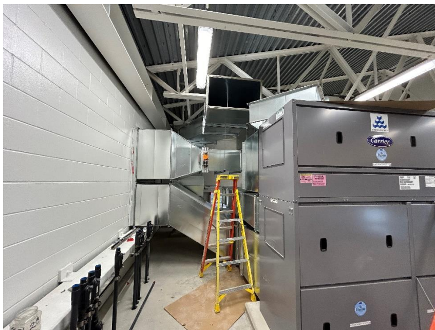
Air handling unit and ductwork at mezzanine level.
