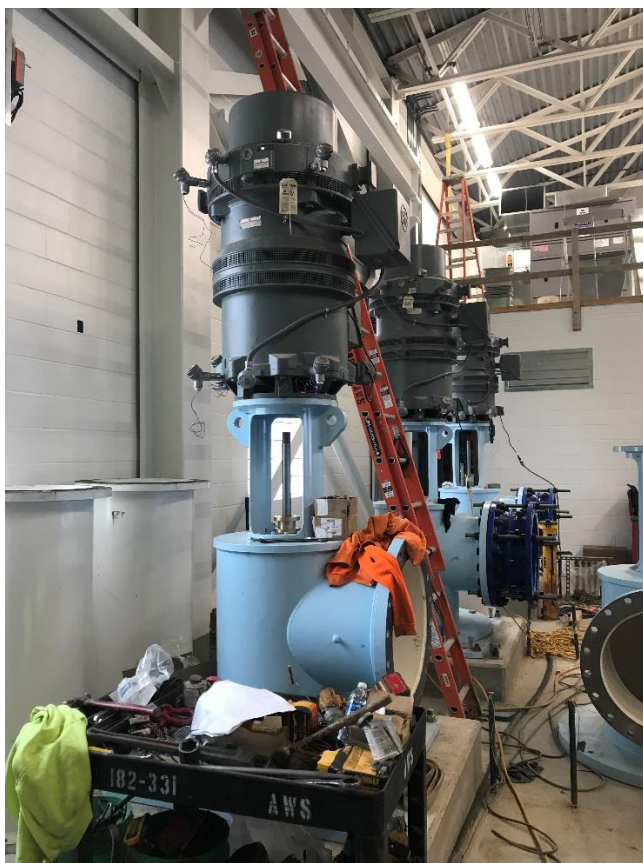
Vertical turbine pump and motor installation.
