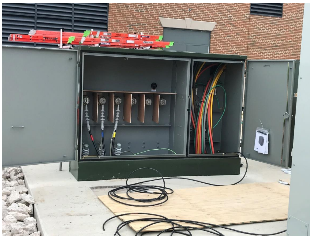
Electrical cable terminations at transformer.
