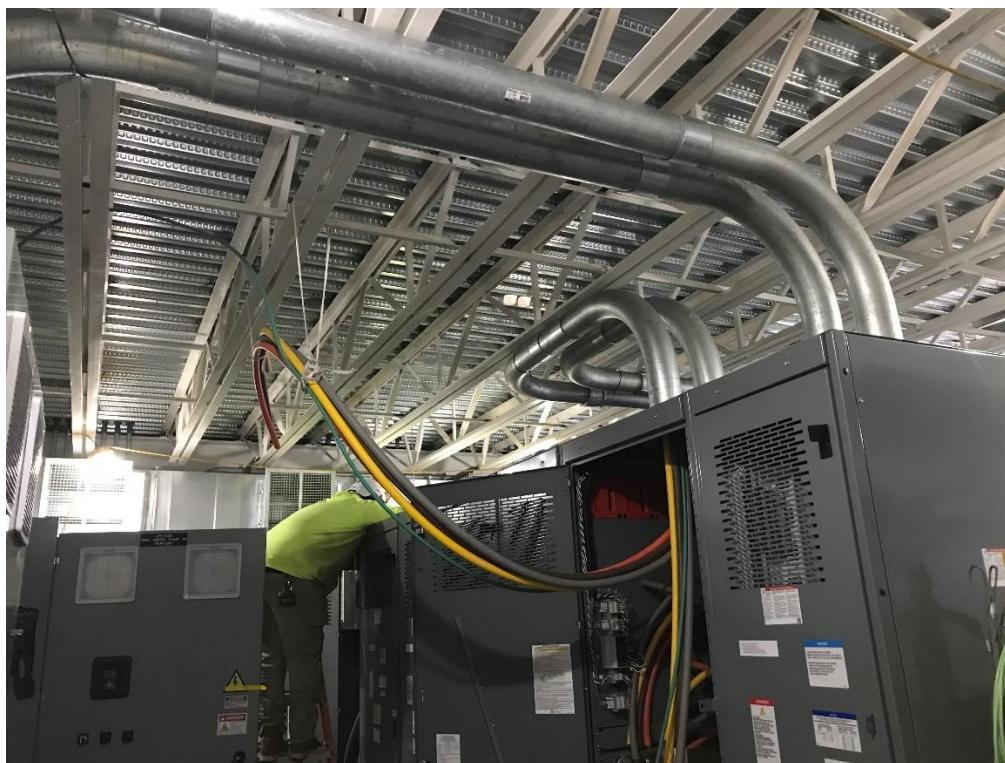
Electrical gear assembly and conduit installation.
