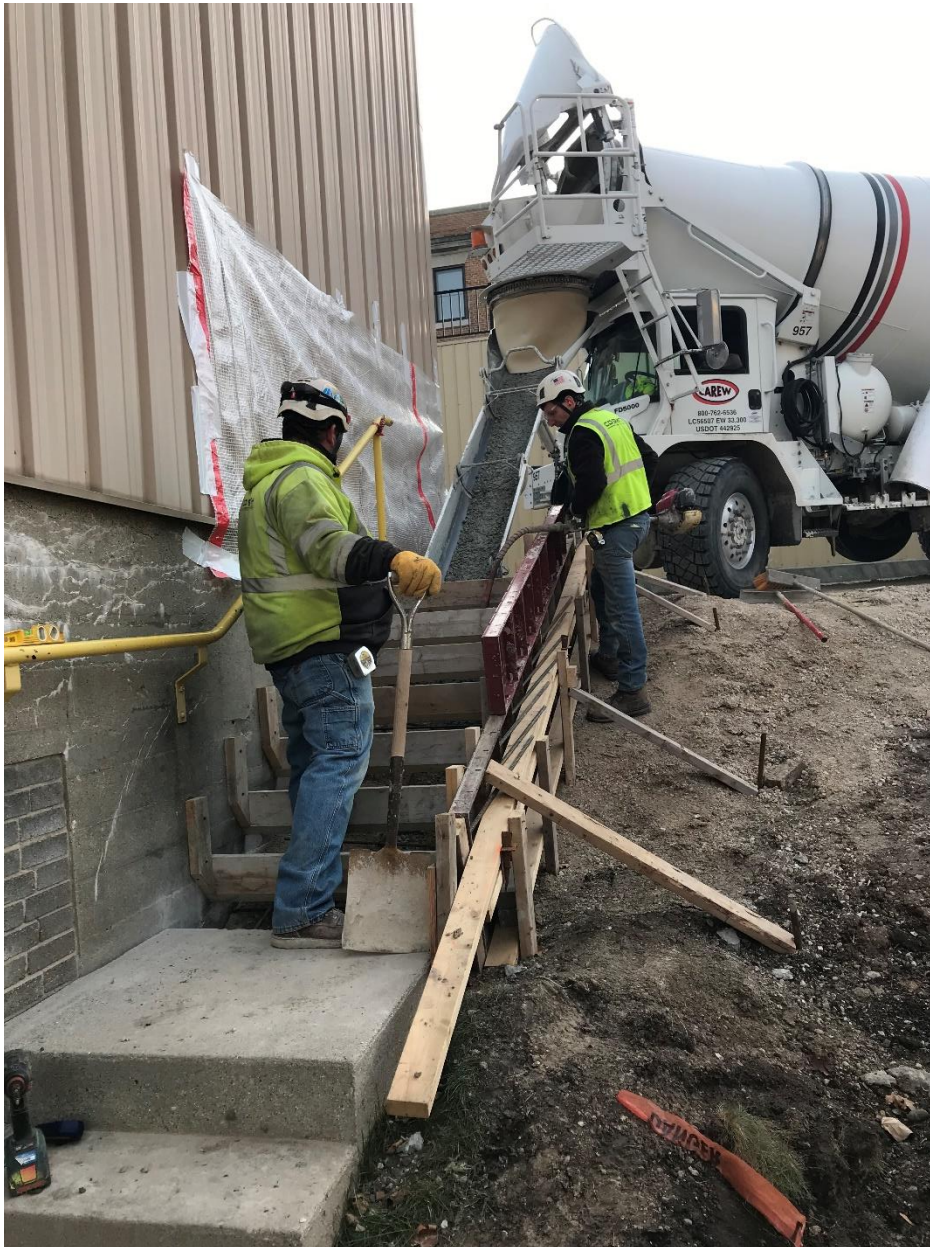
Concrete stair placement adjacent to garage.
