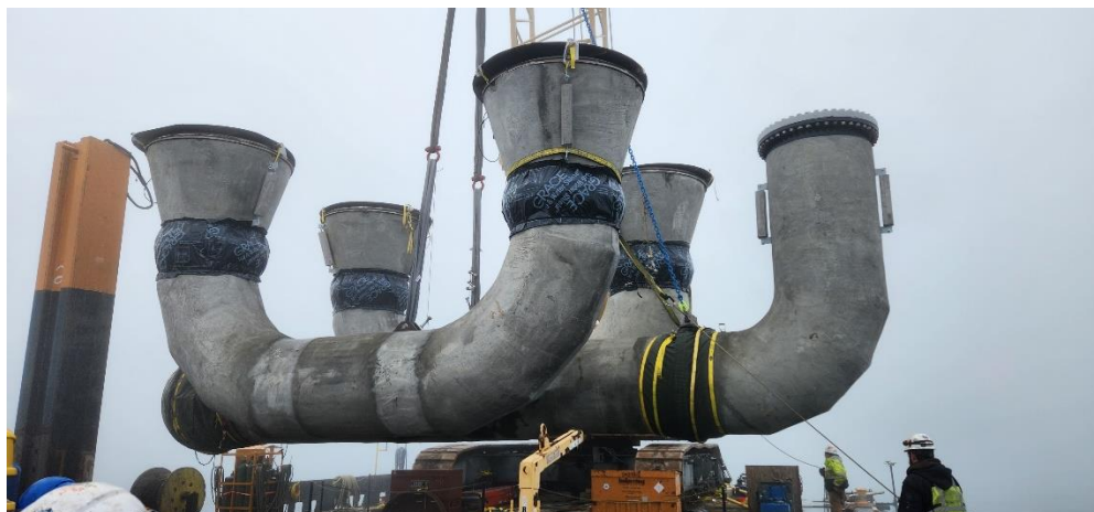
Intake structure lifted off crane barge.
