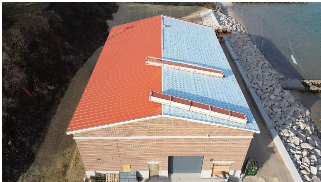
Aerial view of standing seam metal roof installation.
