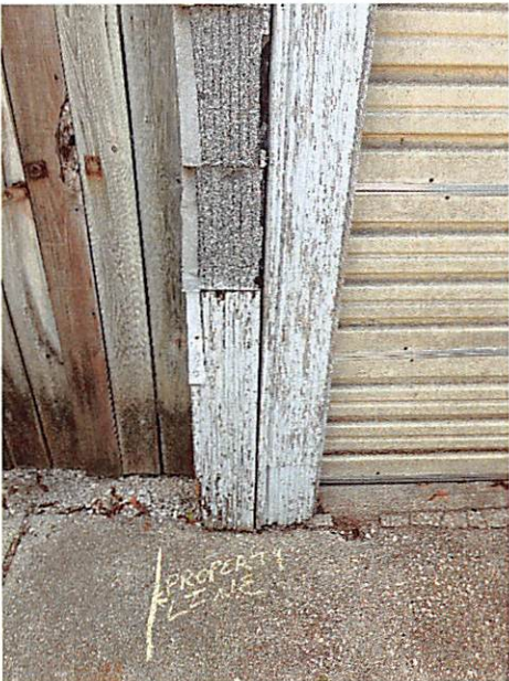
Current garage to North property line
