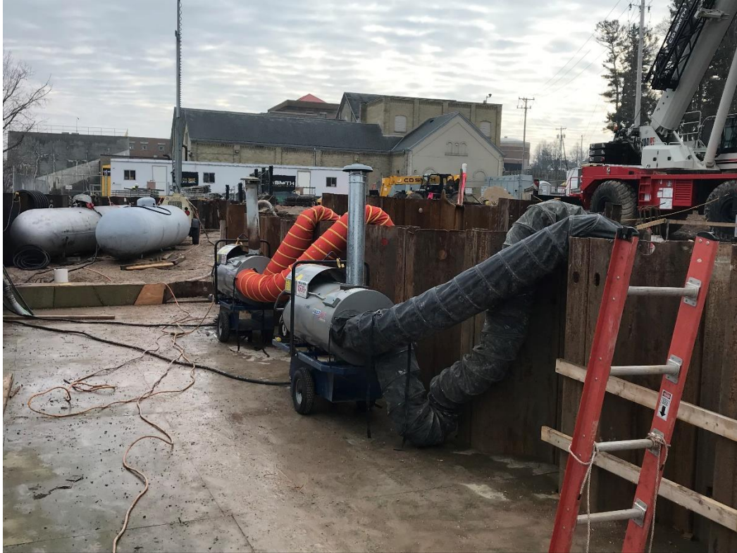
Propane heating system set up for winter concrete.
