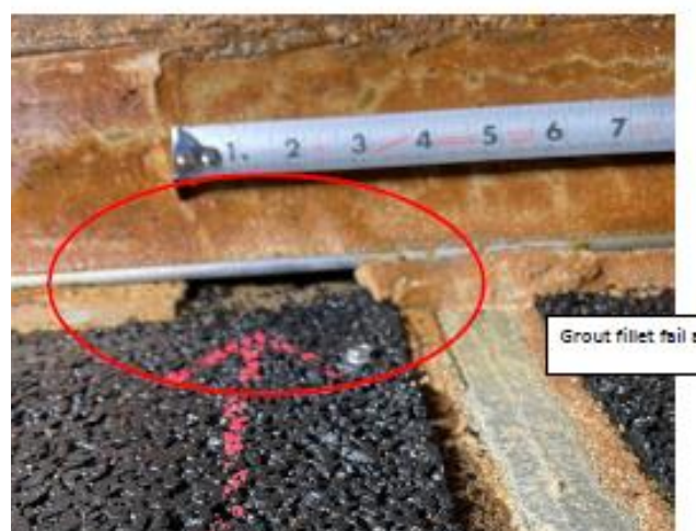
Filter 6 IMS Cap Fail
