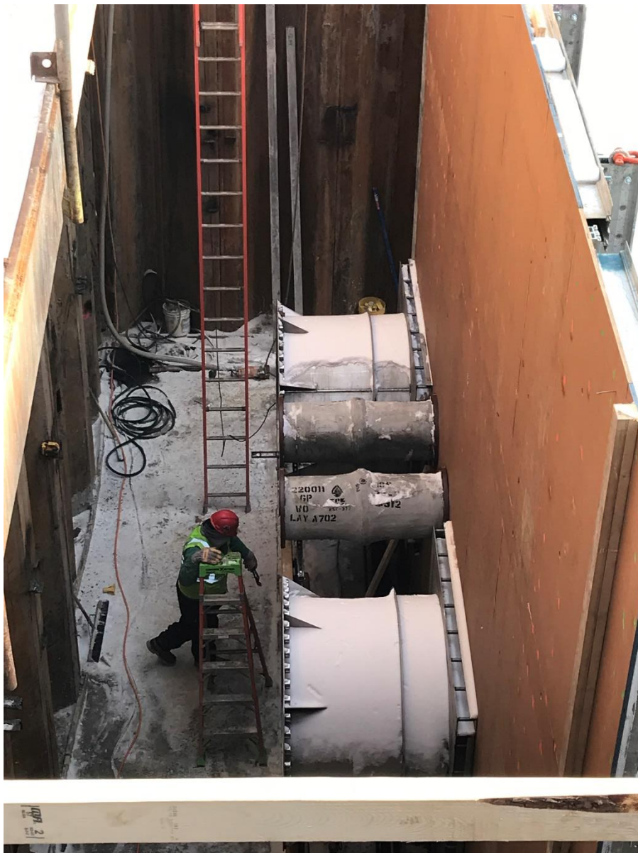
Intake pipe wall thimbles and chemical feed wall pipes set in place.
