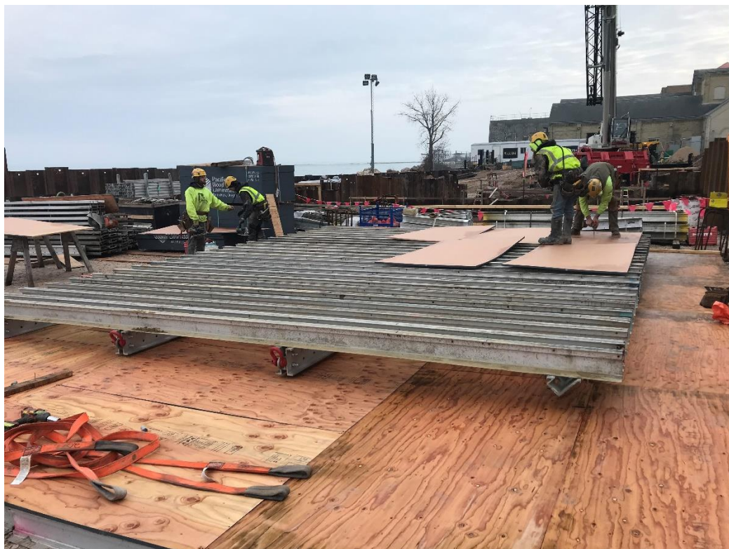
CDS assembles wet well wall form panels.
