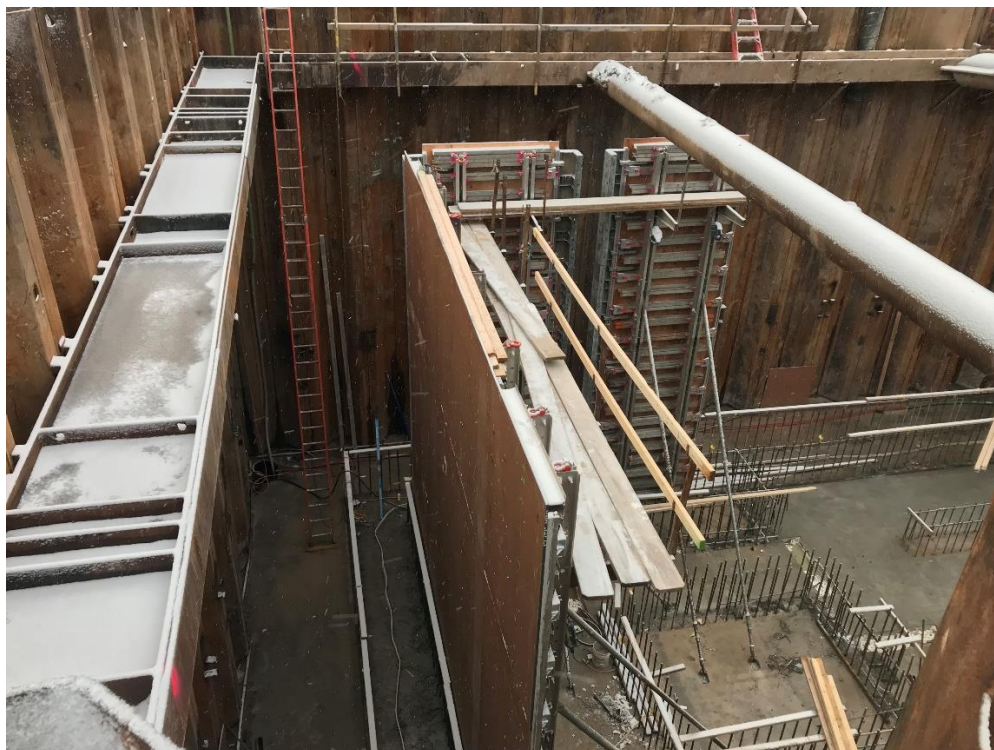
Pump station wet well wall form erection.
