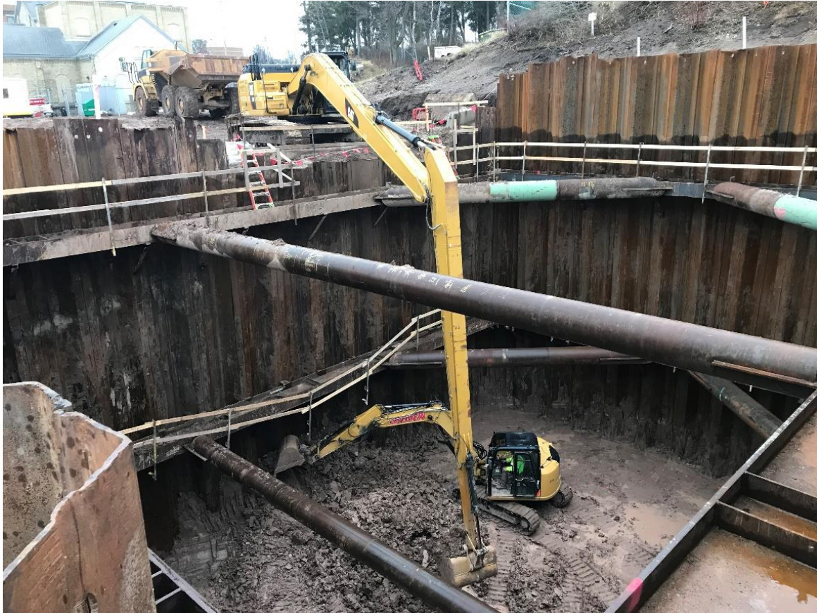
Andrew Excavating completes pump station foundation excavation.
