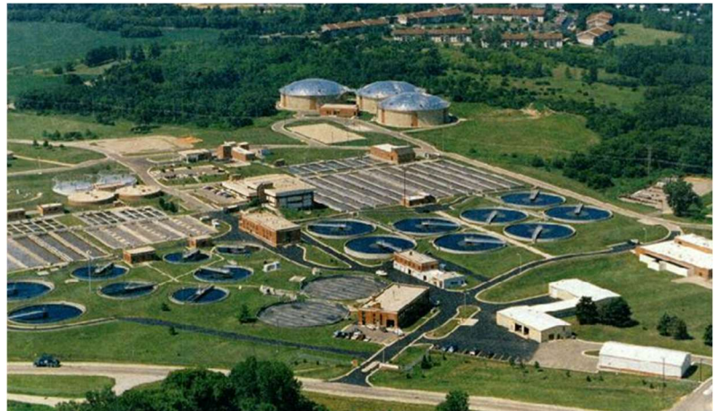
Nine Springs Wastewater Treatment Plant – MMSD.
