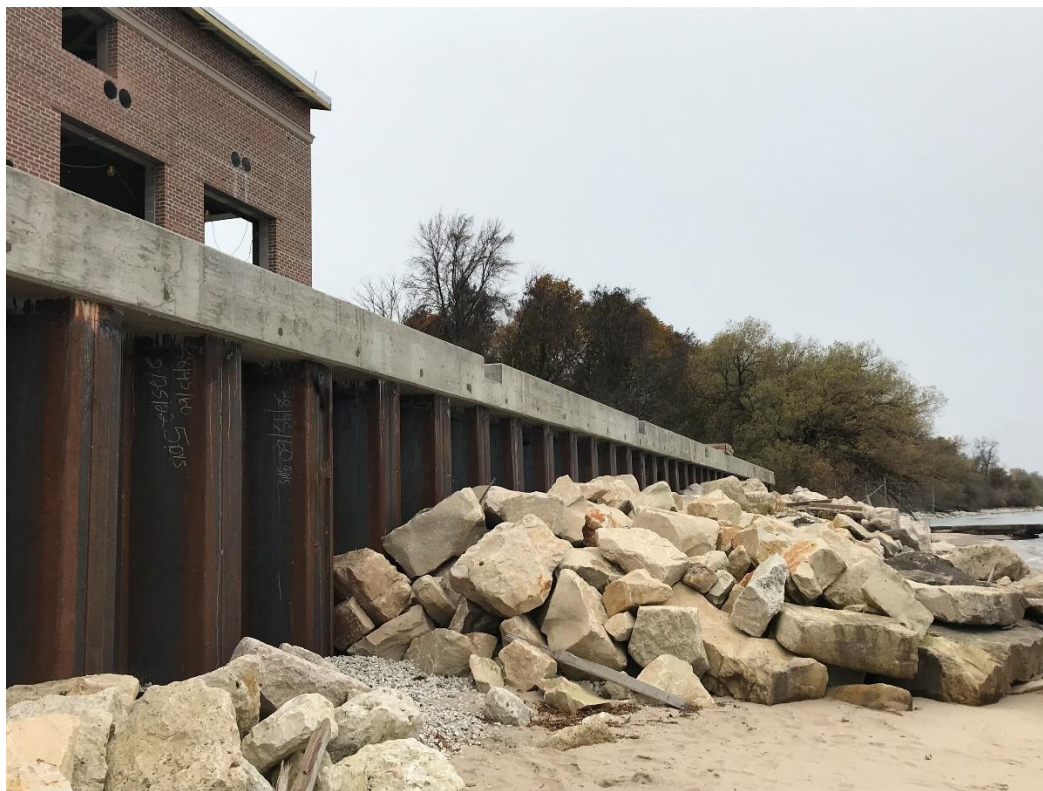
Revetment sheet pile concrete cap.
