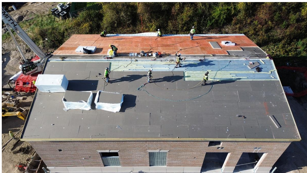
Pump station roof insulation and fire treated plywood is installed.
