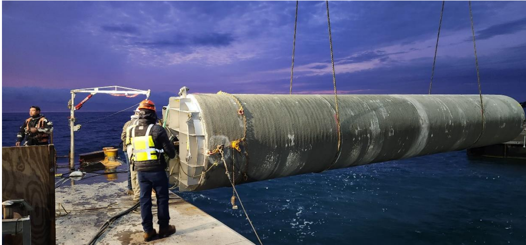
Kokosing prepares main line intake pipe for installation.
