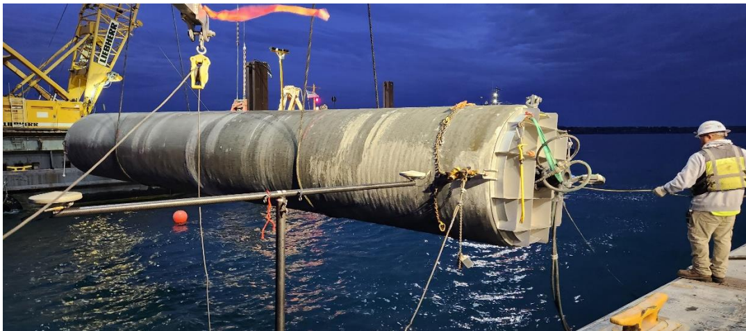
Kokosing installs main line intake pipe.
