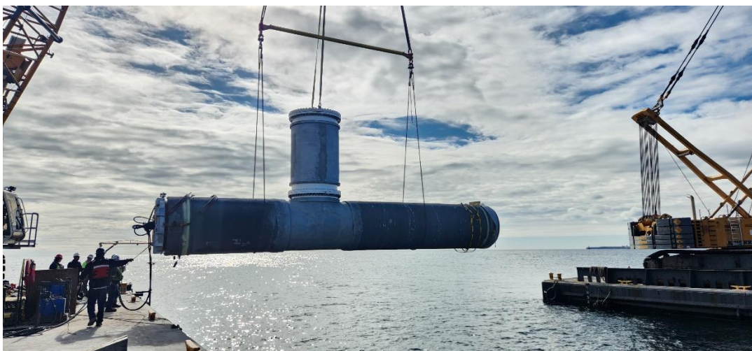
Kokosing installs emergency riser intake pipe section near sta. 50+00.
