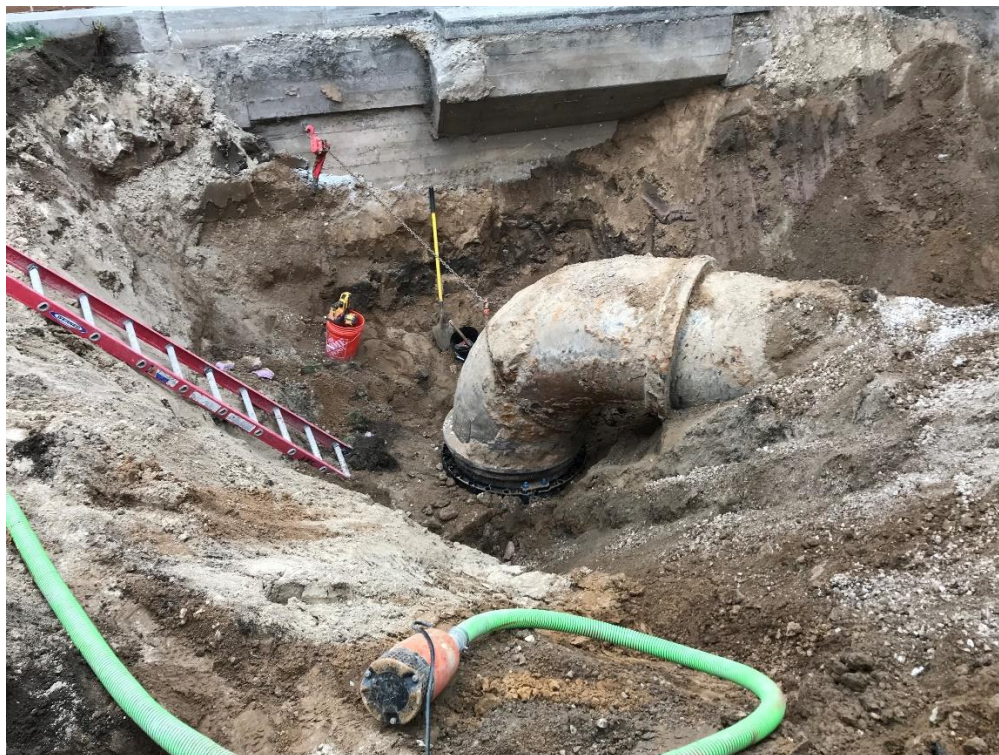
Existing 36" RW pipe exposed at tie-in location.
