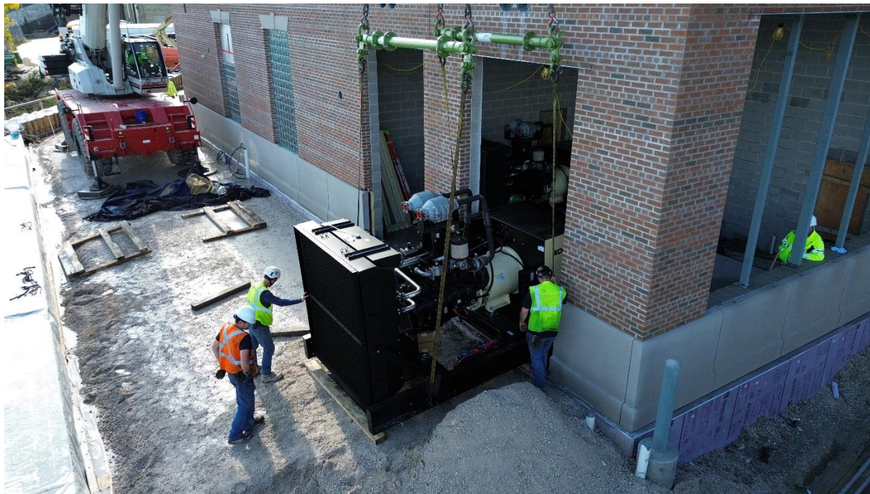
Kohler generator installed through louver opening at pump station generator room.
