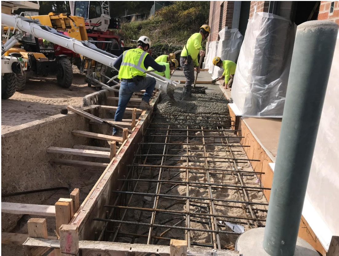
CDS places concrete for south pump station approach slab.
