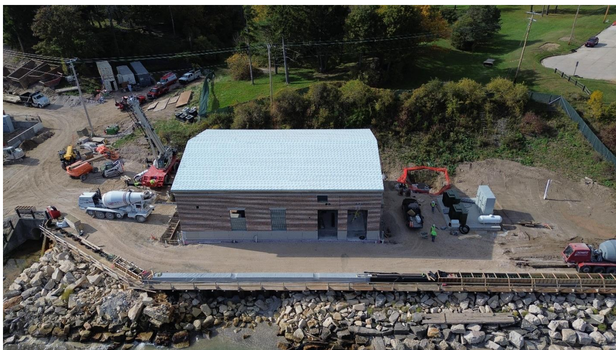
Pump station roof ice and water shield installation complete.
