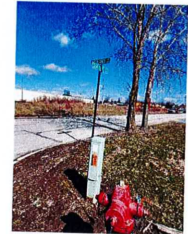
EXISTING FIBER PEDESTAL ④ SCALE: NTS
