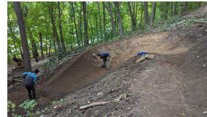
Development of new trails and amenities may require some existing trail re-routes and closures.
