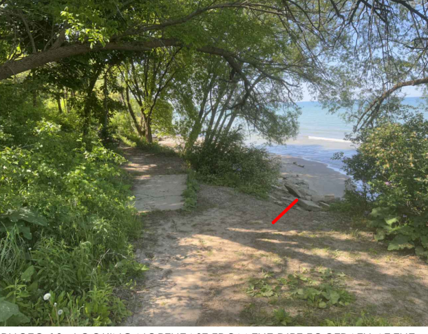
PHOTO 13: LOOKING NORTHEAST FROM THE DIRT FOOTPATH AT THE SOUTHERN END OF THE SUBJECT PROPERTY AT THE EXISTING CONCRETE SLAB TO BE REMOVED. THE RED LINE INDICATES THE PROPOSED LOCATION OF THE SOUTHERN STAIRS.
