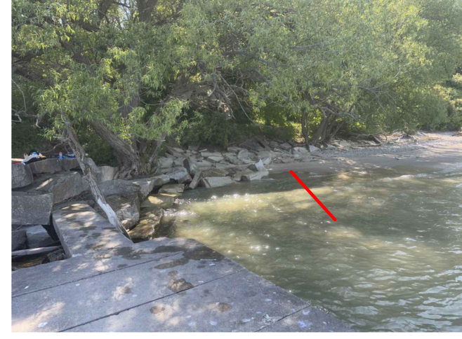
PHOTO 9: LOOKING NORTHWEST FROM THE EXISTING JETTY AT THE EXISTING CONCRETE RUBBLE ALONG THE GRAVEL AND SAND SHORELINE. THE RED LINE INDICATES THE PROPOSED SOUTHERN EXTENT OF THE REVETMENT AND BEACH NOURISHMENT.
