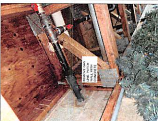
1 EXISTING GENERATOR GAS PIPING E1.2 NTS
