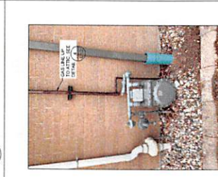
1 EXISTING GENERATOR GAS PIPING E1.2 NTS
