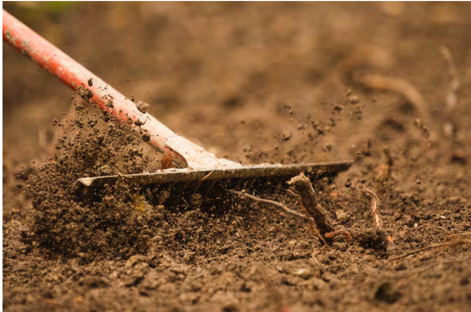
Trail construction employs a host of advanced tools, but sometimes the job simply calls for the time-tested rake.
