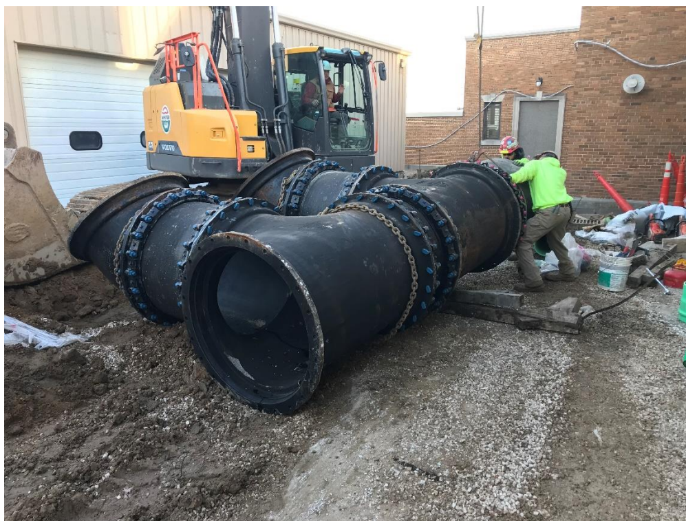
36" RW pipe assembled for tie-in.
