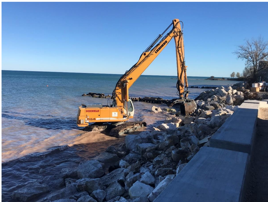
Michels installs revetment stone.
