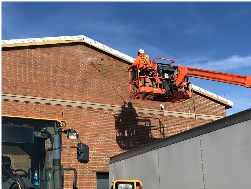
Pump station face brick washing.
