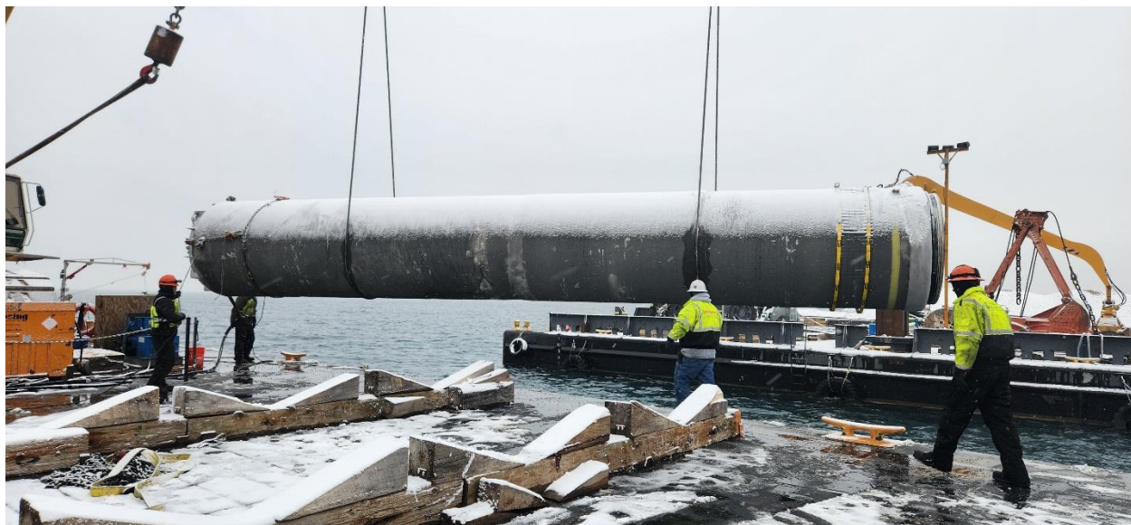
Kokosing prepares to install intake pipe.
