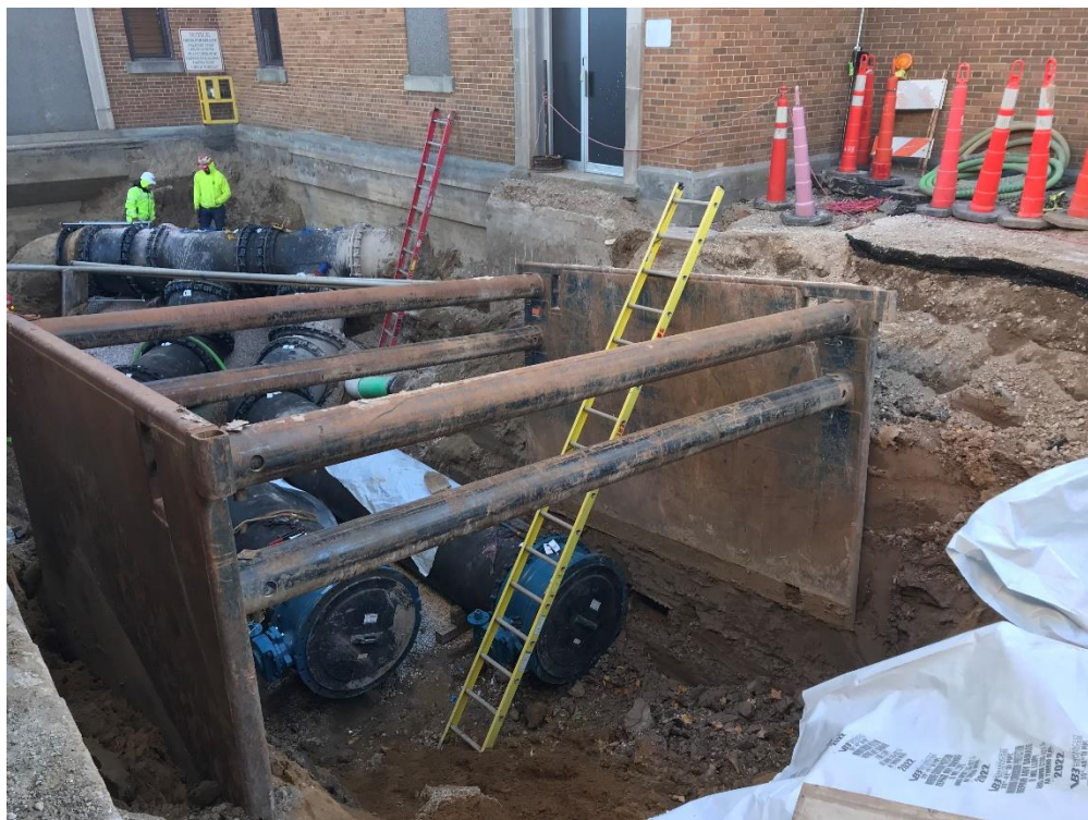
36" RW pipe installed at tie-in location.
