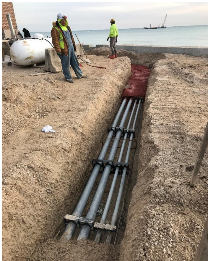
Electrical ductbank concrete placement.
