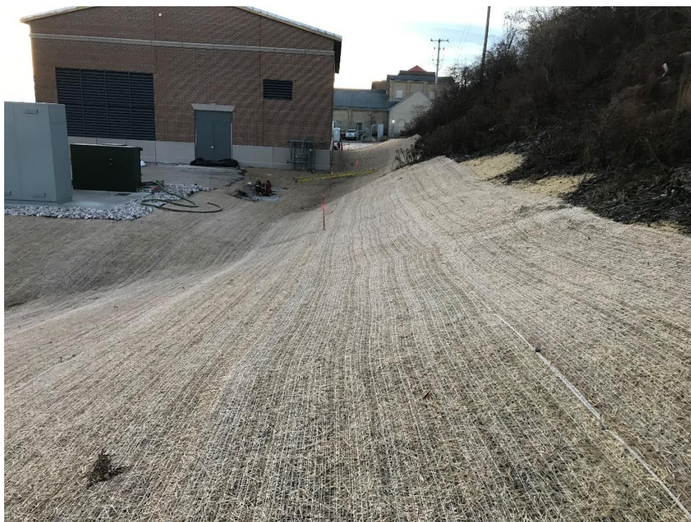
Seed and erosion control mat placed north and west of pump station.
