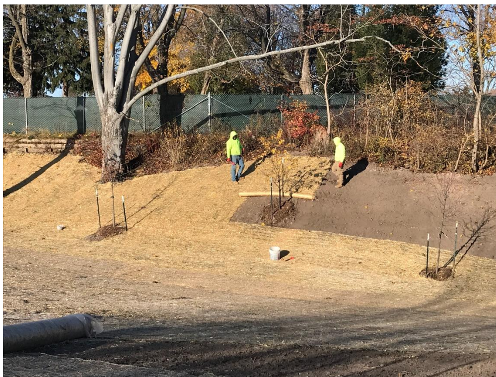
Seed and erosion control mat installed in ravine.
