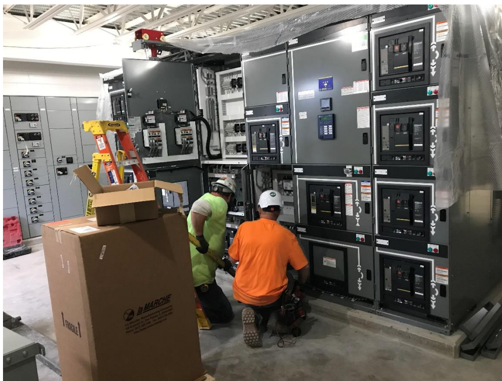
Electrical gear installation.
