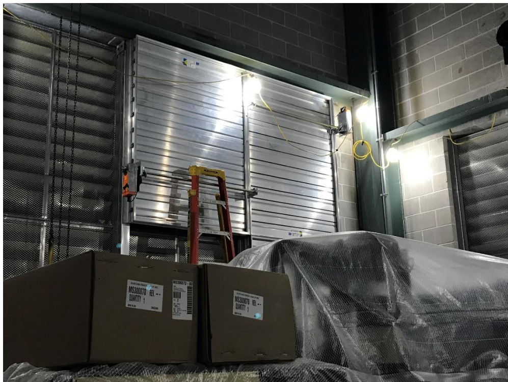
Louvers and dampers installed in generator room.
