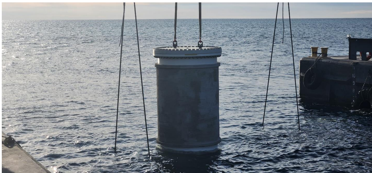
Kokosing installs final emergency riser section at sta. 60+00.
