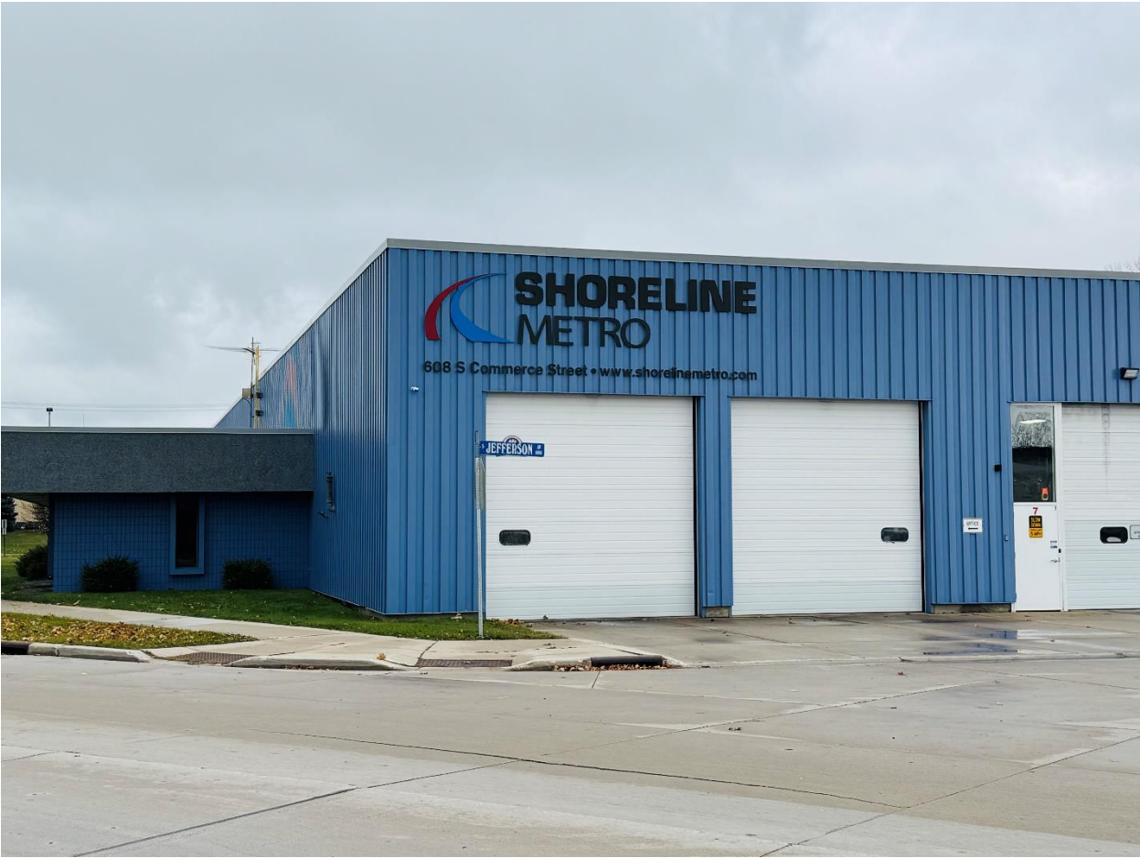
Exterior view of the Shoreline Metro administration and maintenance facility.
