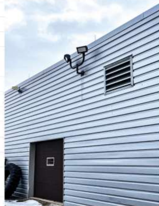
Exterior security lighting at the Sheboygan Police Department
