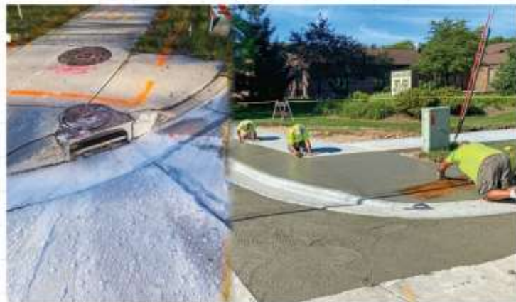
ADA-compliant ramp installation
