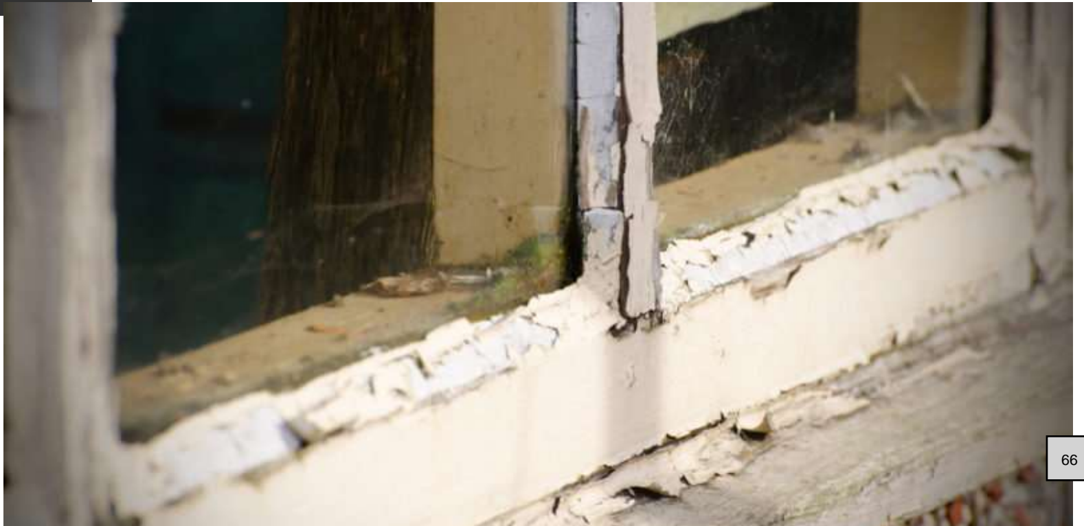
Lead-Based Paint on Windows
