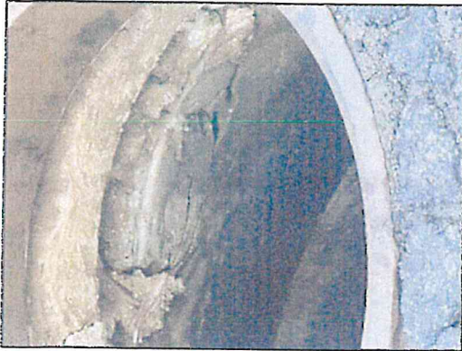
MH 101, cone damage
