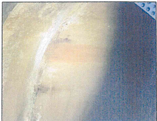
Image 6 – Cone and barrel section infiltration
