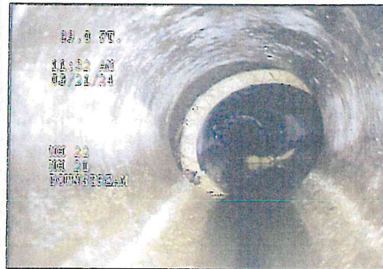
MH 22 to MH 21, offset at joint
