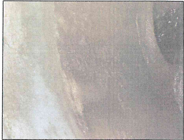
Image 4 – Connection 2, joint infiltration
