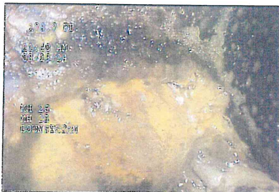
MH 26 to MH 25, infiltration runner
