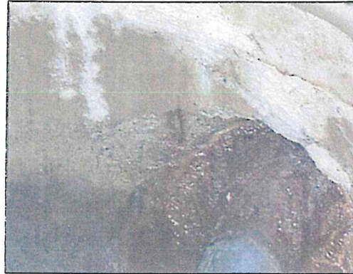
MH 105, exposed rebar
