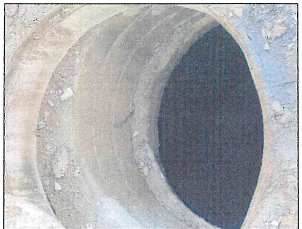
Image 4 – Chimney and Frame offset
