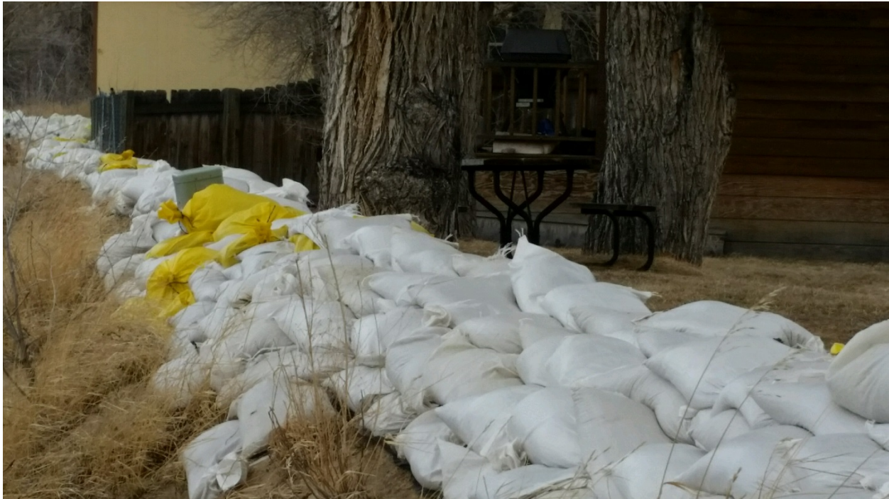
Photo No. 5 – View of 2016 sandbags that are still in satisfactory condition.
