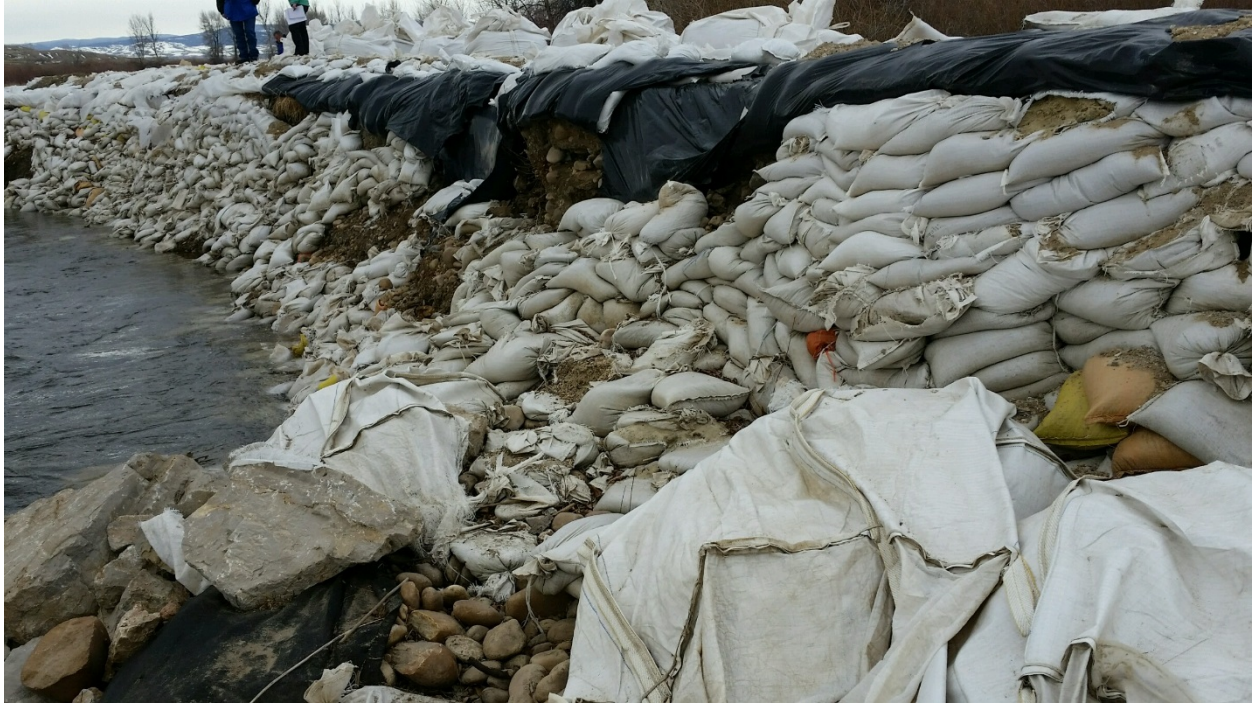
Photo No. 4 – View of the upstream face of the embankment, from near the upstream culvert, looking upstream. Note the vertical embankment face, deteriorating sandbags, and exposed embankment material.
