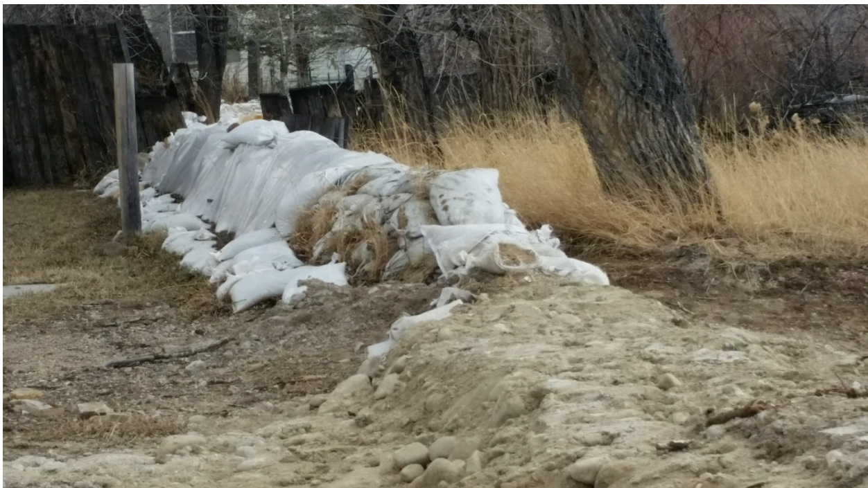
Photo No. 6 – View of 2016 sandbags that are badly deteriorating, and an adjacent area where a portion of the sandbags have been removed.
