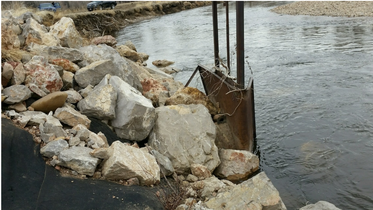
Photo No. 1 – View of the intact, downstream headgate. Riprap on the riverside face starts at this location on the embankment.
