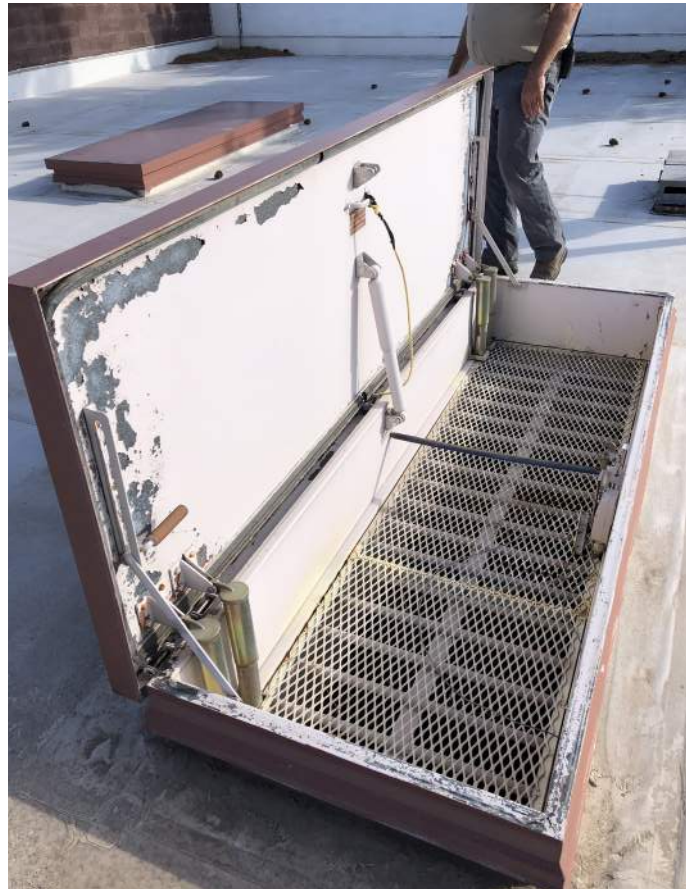
pictured: photo of existing secured skylights above dorm rooms
