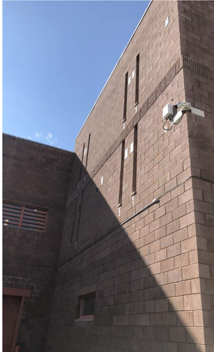
pictured: photo of existing masonry exterior and dorm room openings
