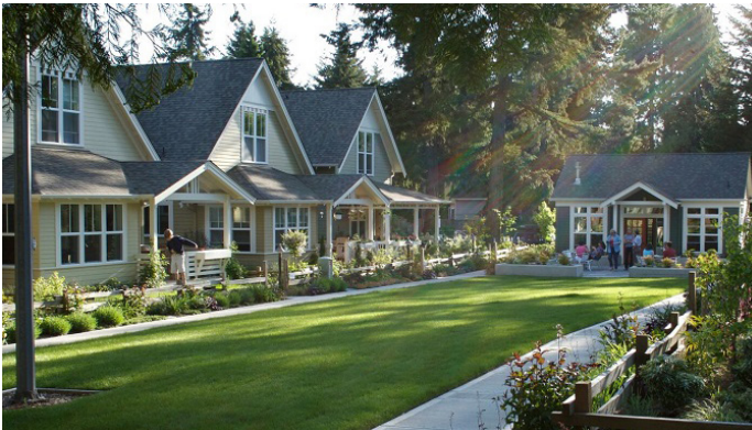
Yard Buildings - Garden Court
