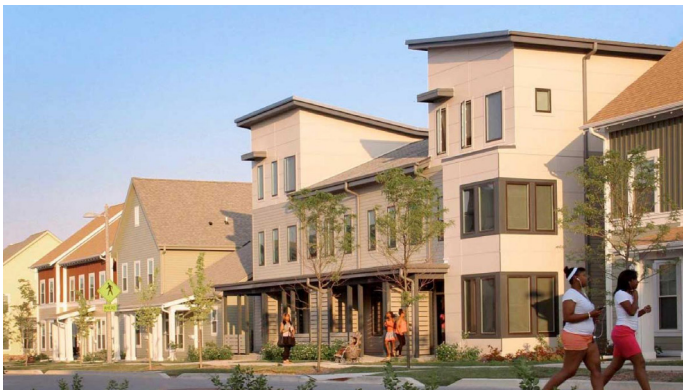
Row, Yard, and Stoop Buildings - a Mixture of Building Types
