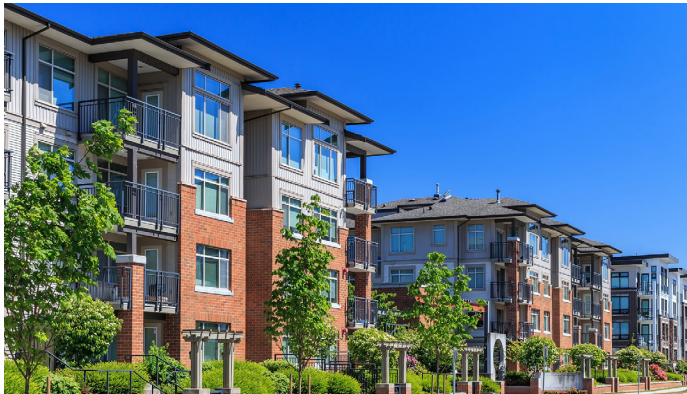
Stoop Building - Mid-rise Multi-family Residential
