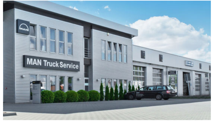
Limited Bay Building - Commercial
