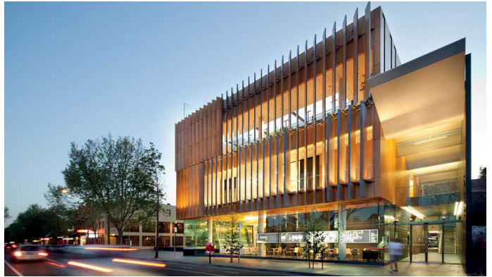
Civic Building - Performance Space
