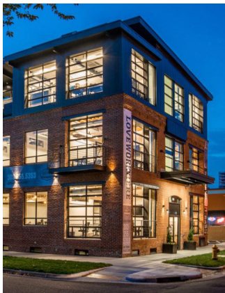
Primary Materials: Brick
