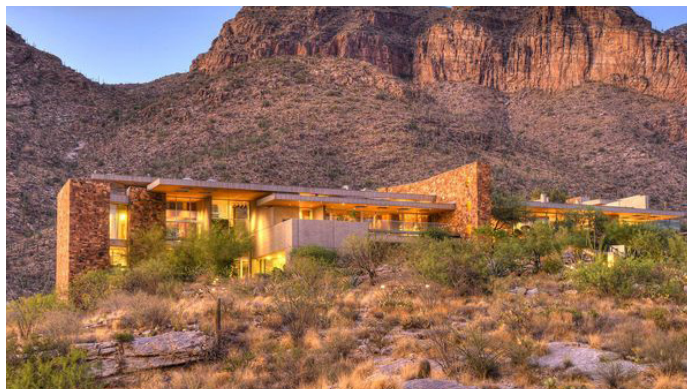
Yard Building - Large-Lot Single-Family
