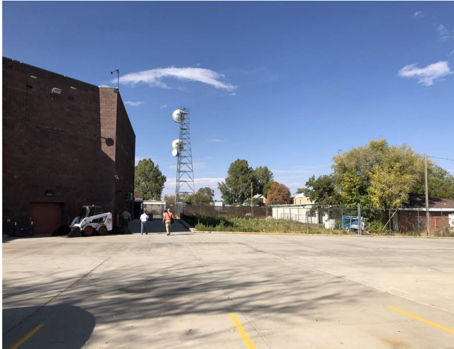
pictured: photos of the existing public safety building
