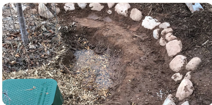
Installing earthworks for a gravity-fed graywater system in Moab, UT (pipe outlet into green mulch shield). Credit - Roslynn Brain McCann
