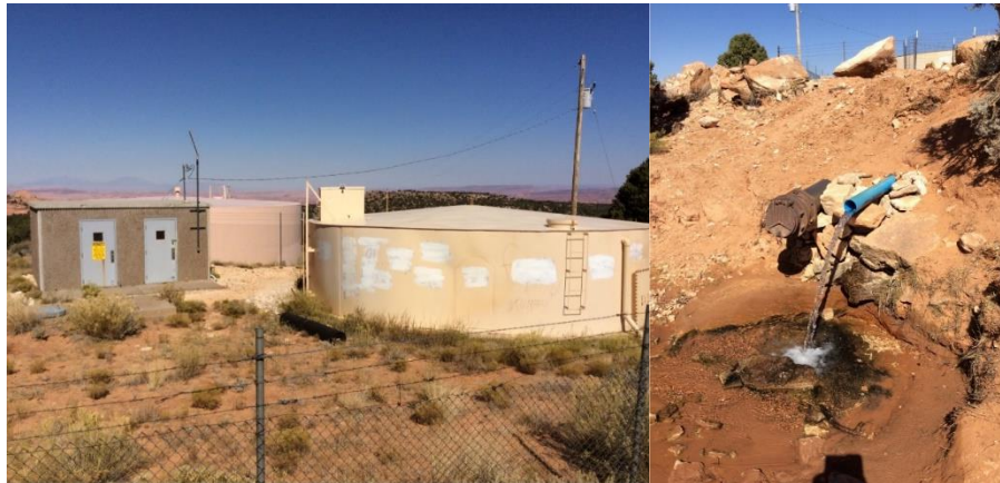
Figure 1. Existing 50,000 Gallon Tank and overflow to nearby creek
