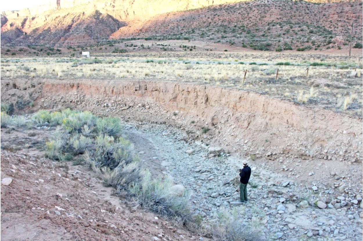
Figure 3-1. Pack Creek Channel in Valley Floor
