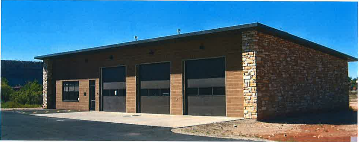
Bluff Fire Station Completed in 2006
