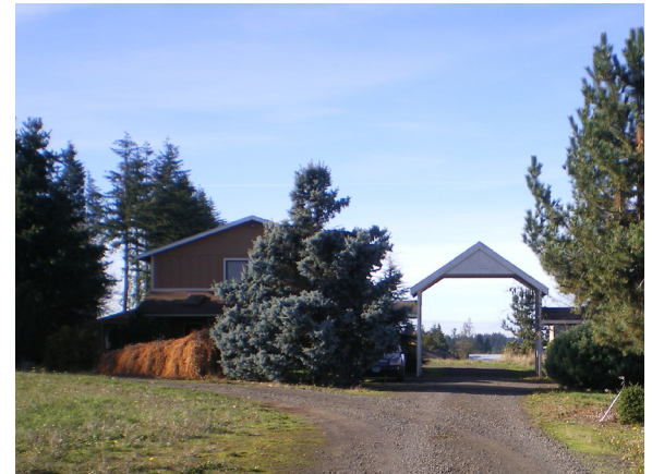
Existing Bunk House to be Removed
