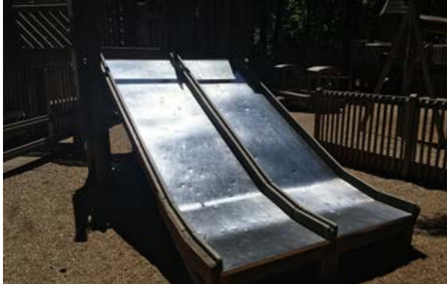
2. Deteriorating slide with loose composite sideboards
