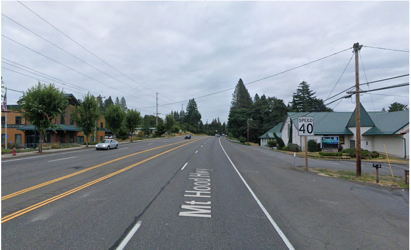
(1) Looking east from 200 feet east of SE Ten Eyck Road.
