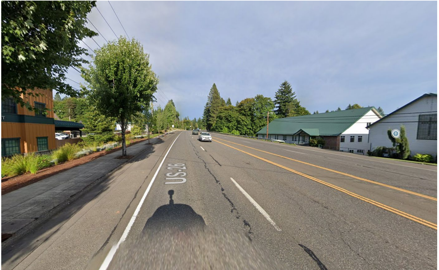
(3) Looking east from 300 feet east of SE Ten Eyck Road.
