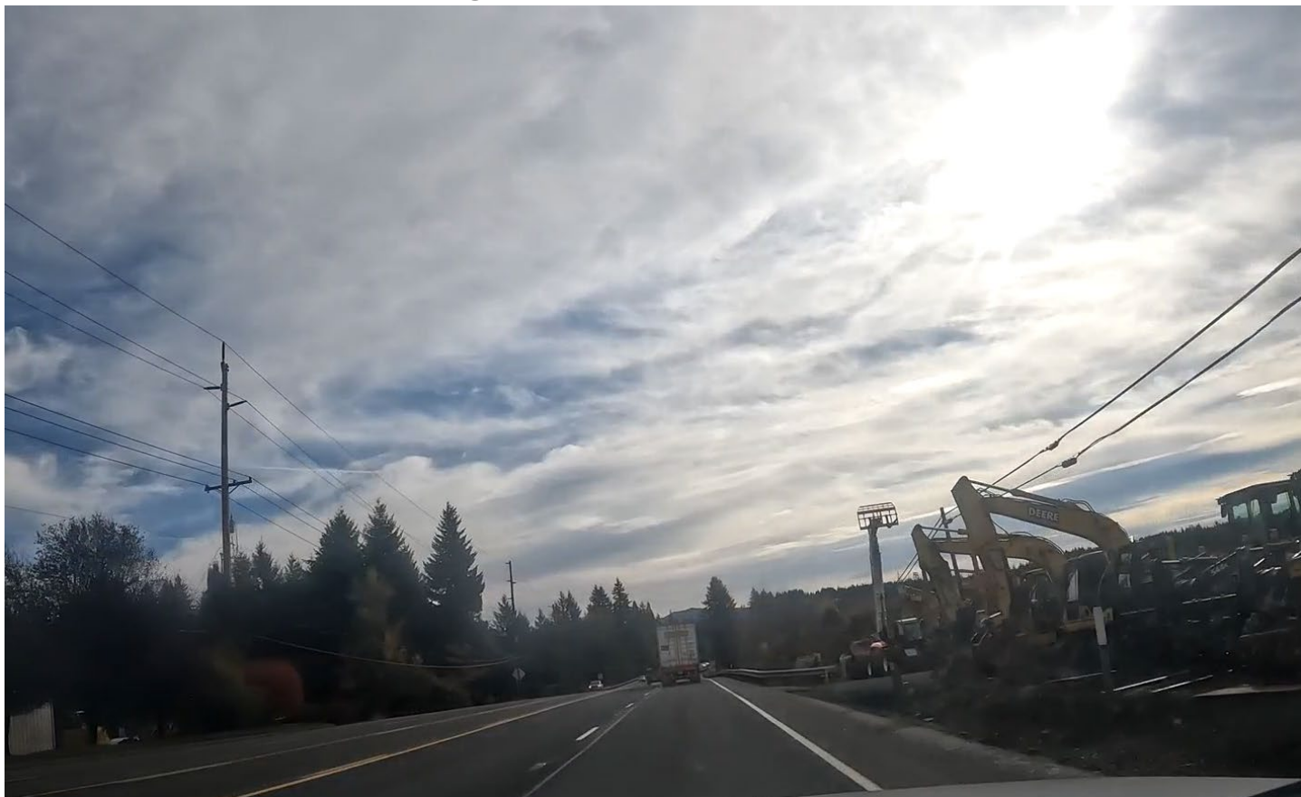
(13) Looking east from 0.22 mile west of SE Canyon Valley Road.
