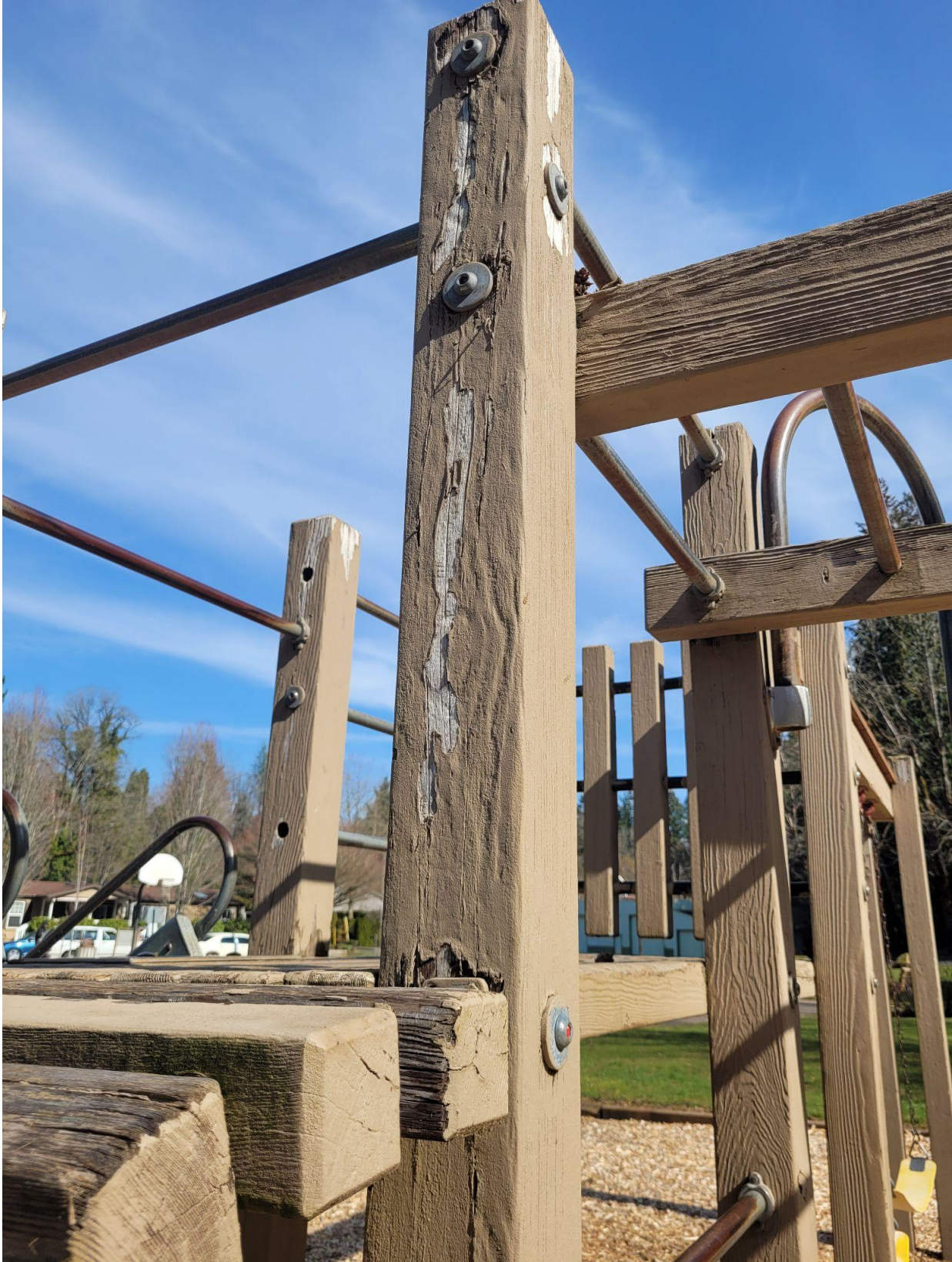
Tupper Existing playground structure:
