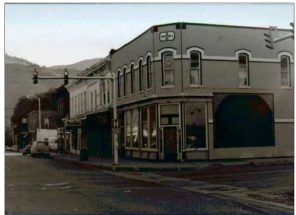
Photo 7: Twitchell Building, 101 N. F Street (5CF.406.45).
