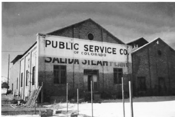
Photo 40: Edison Electric/Salida Steam Plant (5CF.291)
