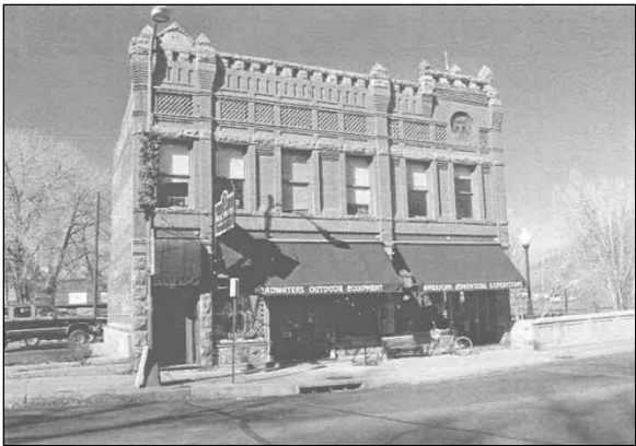
Photo 16: Bon Ton/Manhattan Hotel, 228 N. F Street (5CF.213)..
