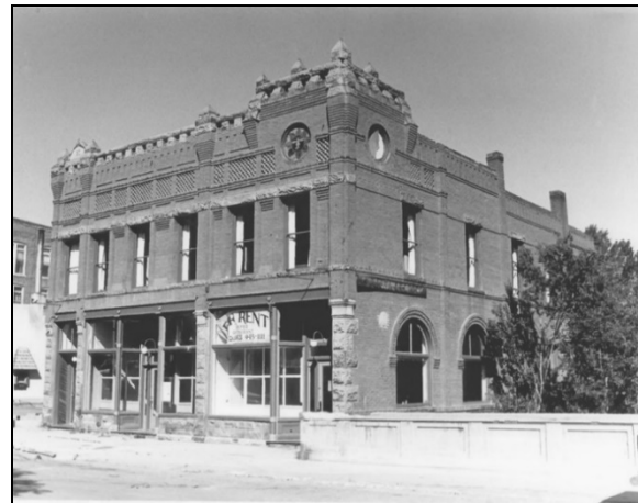
Photo 46: Manhattan Hotel (Source: NR Nomination)
