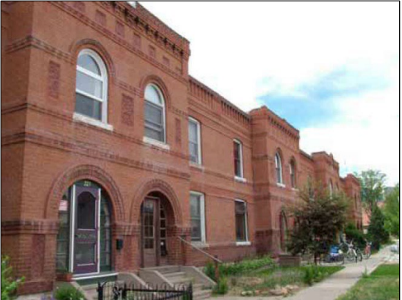
Photo 27: Comstock Terrace, 223-249 E. Street (5CF.2247) was found potentially Eligible to the NRHP.
