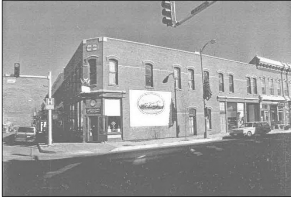
Photo 14: Twitchell Building, 101 N. F Street (5CF.406.45).
