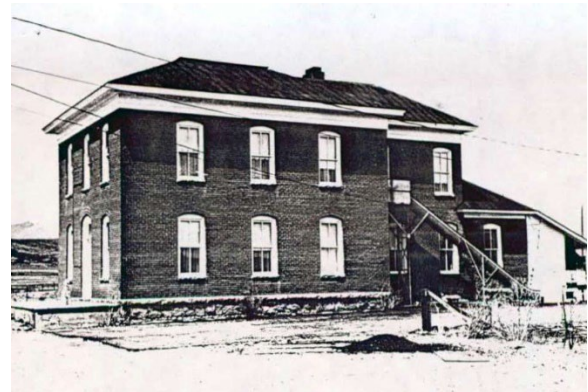
Photo 31: Chaffee County Poor Farm (5CF.190)
