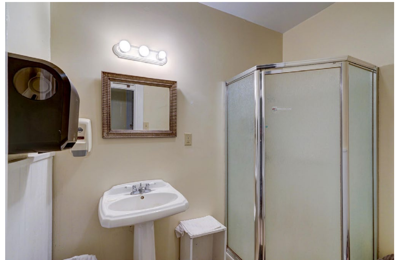
Existing shower for entire hotel space - to become laundry room
