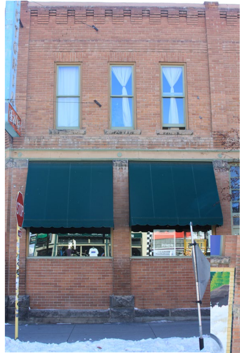
F Street brick infill windows
