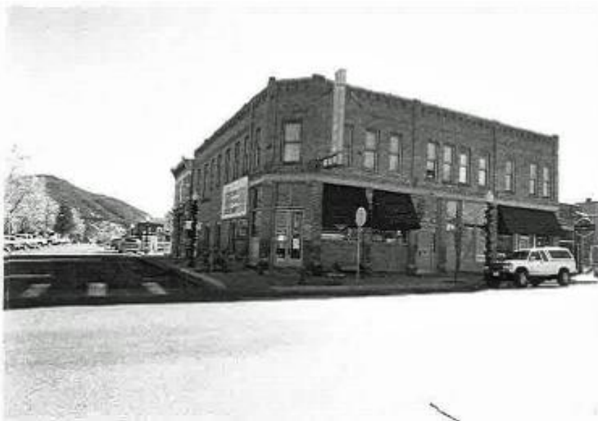
Four photos of the Victoria Tavern taken during the re-survey of the Downtown Historic District 2001-02 . From North F Street\ Colorado Cultural Resource Survey – Architectural Inventory Forms\The Salida Archive\, courtesy Salida Regional Library.
