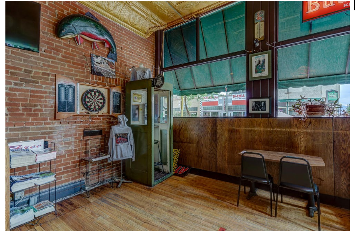
Interior Bar brick walls, floor and interior plywood at F Street window infill
