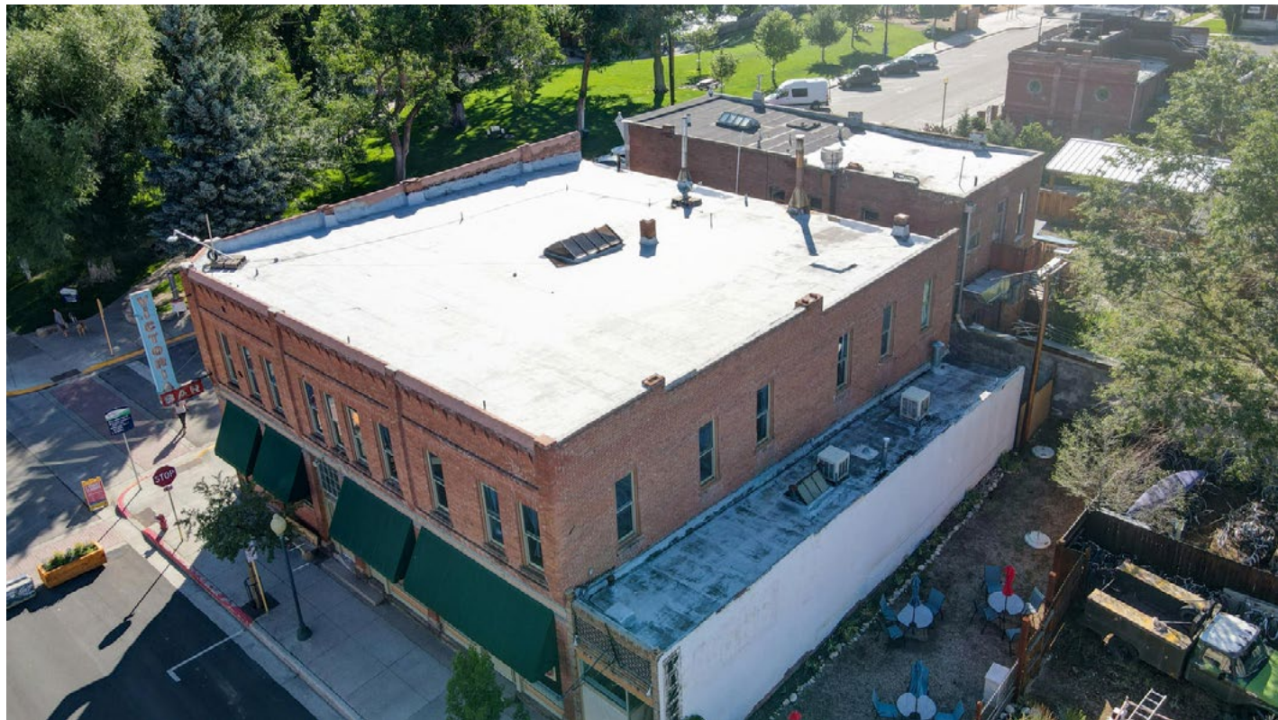
Roof View including one-story Cafe
