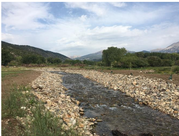
Stabilized river bank to the river
