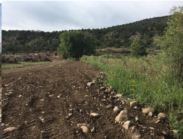
Backfilled wetlands that lead
