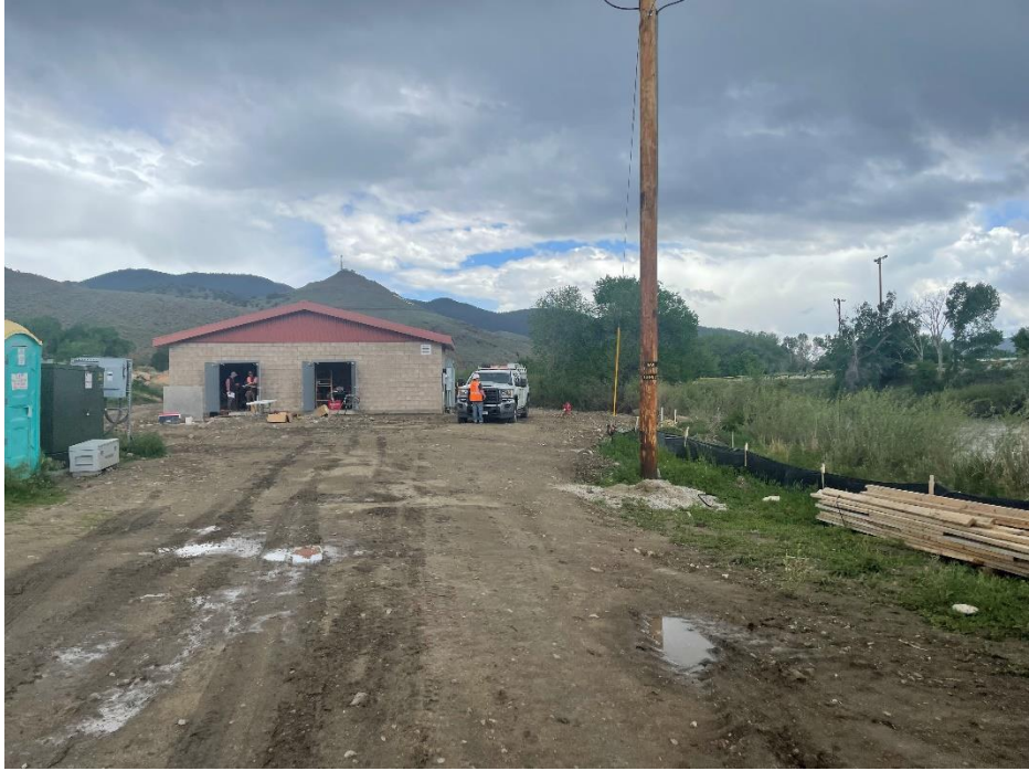
Figure 1 - Pump Station Building
