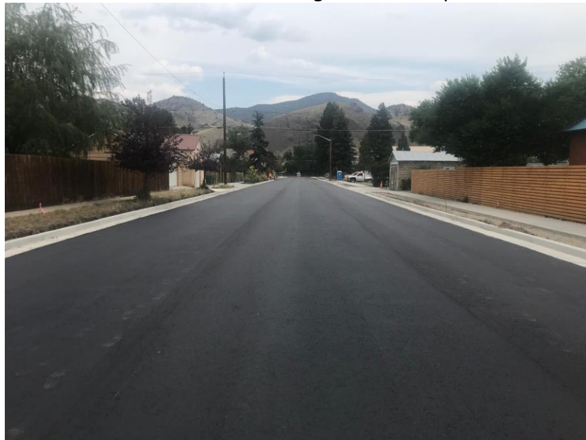
Figure 1 - B Street Reconstruction
