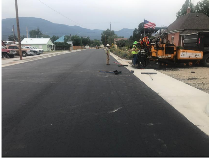
Figure 2 - B Street Reconstruction
