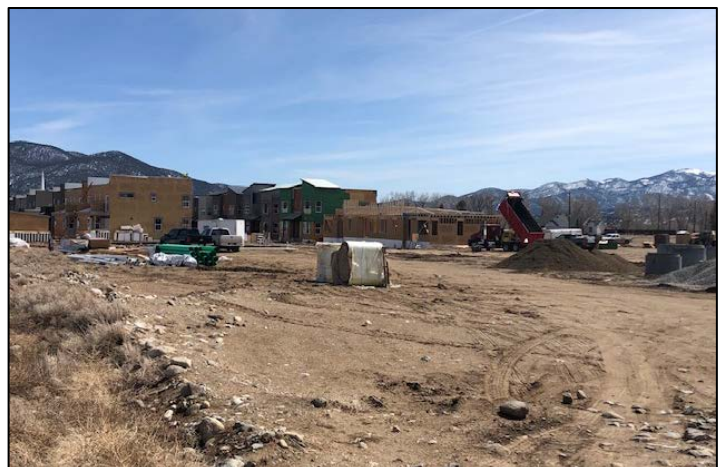
Close-up of multi-family development to the S/SE (City)
