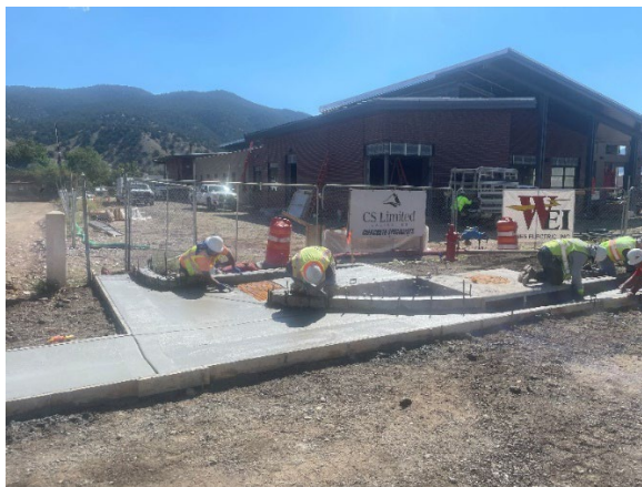
Oak Street Curb and Sidewalk Fronting Fire Station
