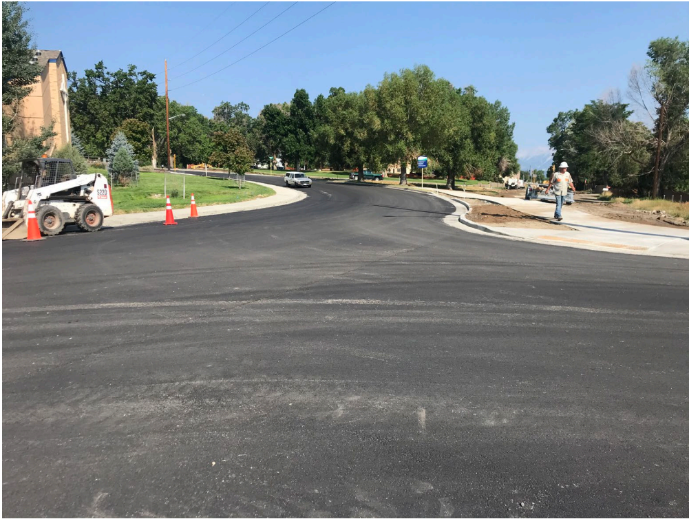
Figure 2 – Poncha Blvd and 3 rd St. Improvements
