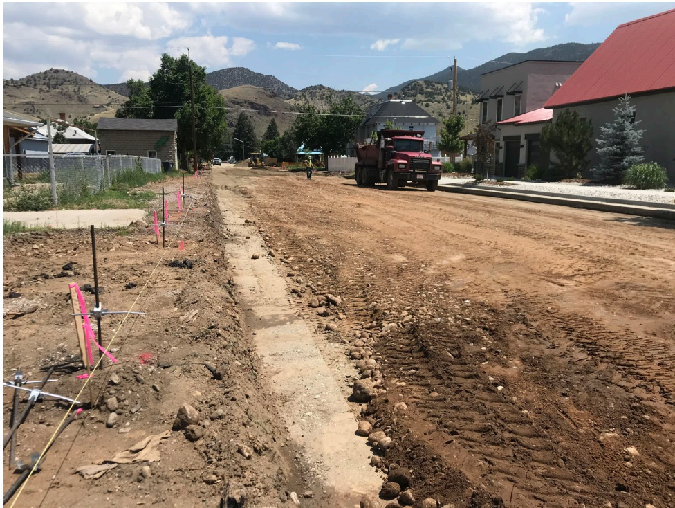
Figure 3 – B Street Reconstruction
