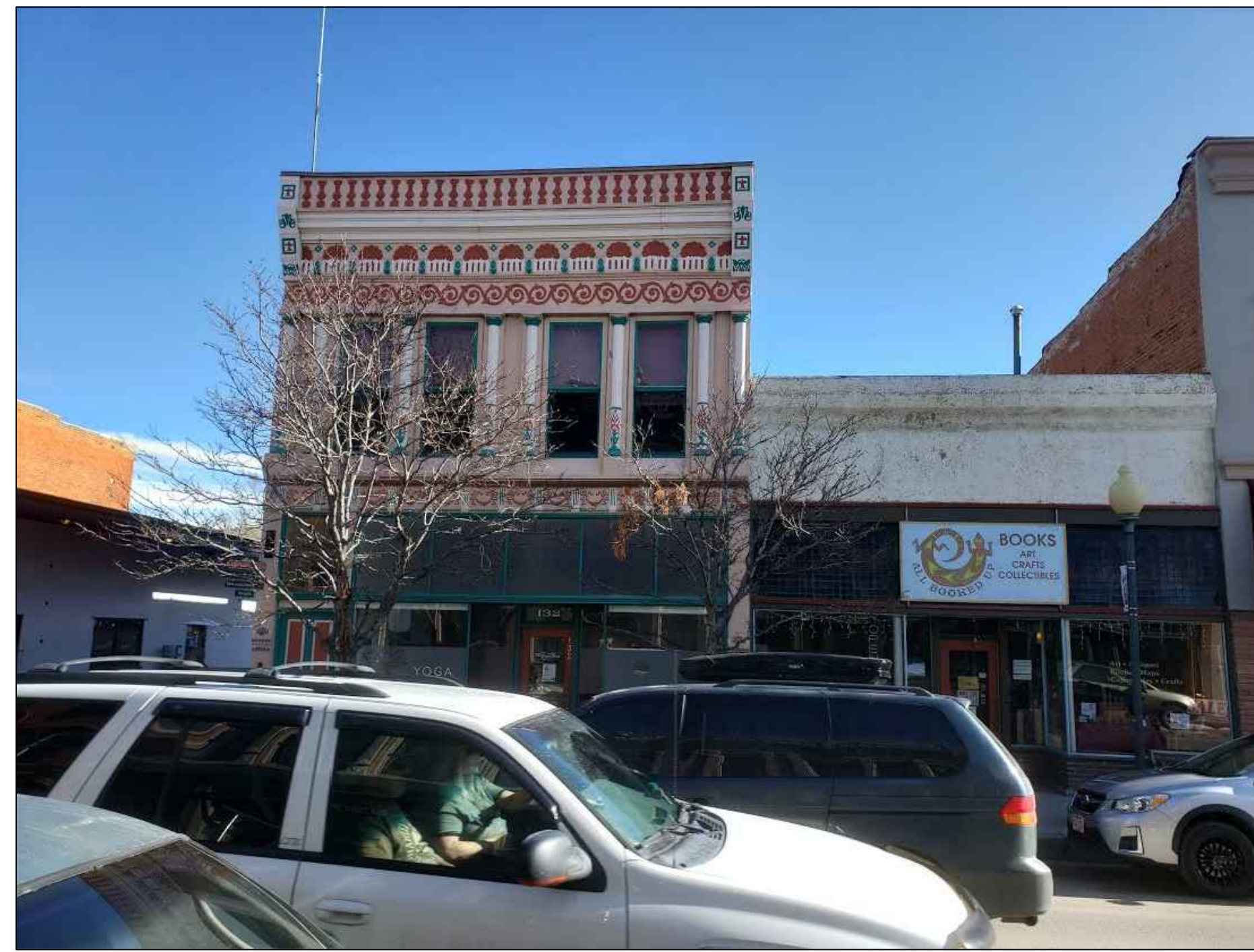
SUBJECT PROPERTY 128 E. FIRST STREET
