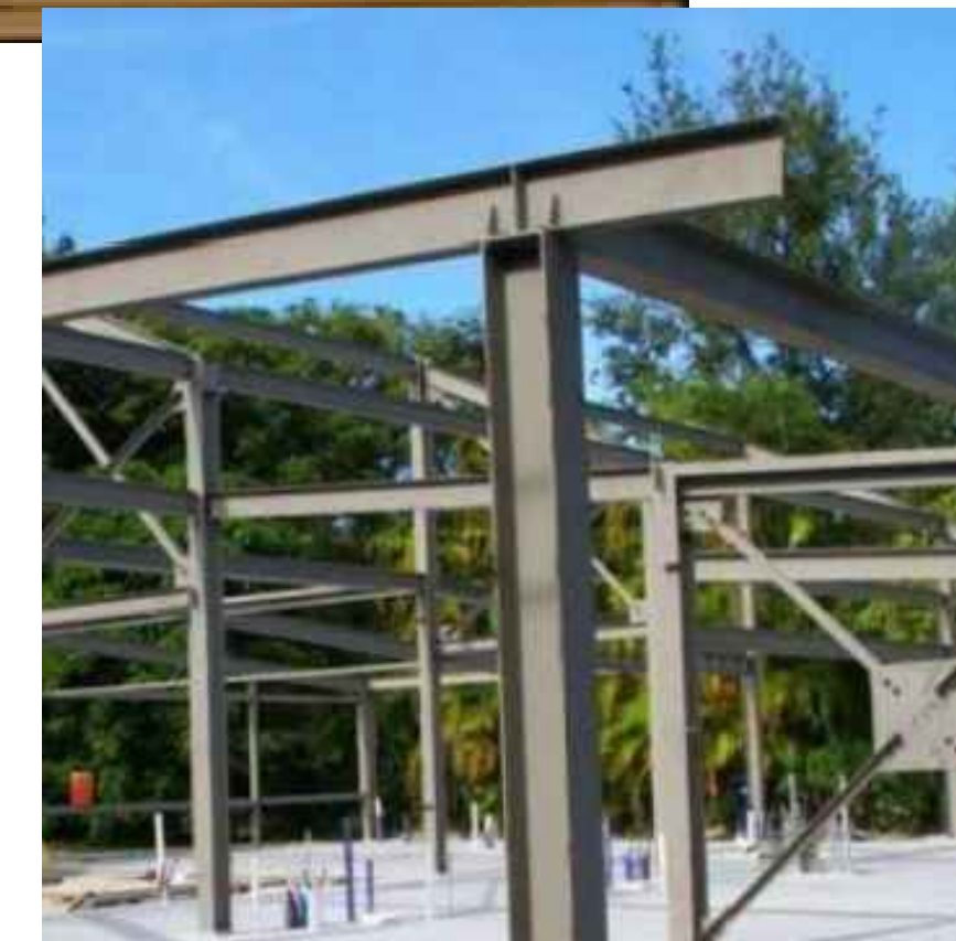
EXPOSED STRUCTURAL STEEL FRAME AT GROUND LEVEL
