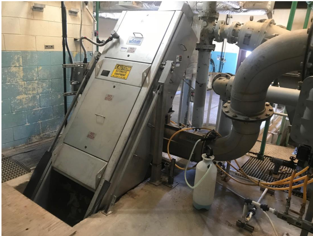
Figure 1 – Bar Screen Replacement
