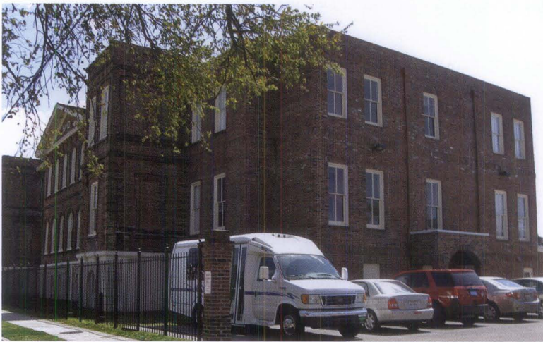
Figure 9. A simple, brick stair tower replaced two non-historic additions at the rear of this 1879 school building when it was rehabilitated as a women's and children's shelter. The addition is set back and it is not visible from the front of the school.
