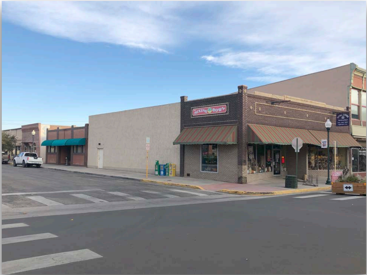
Corner of 2nd and F Street showing neighboring building 148 F Street and 120 West 2nd Street
