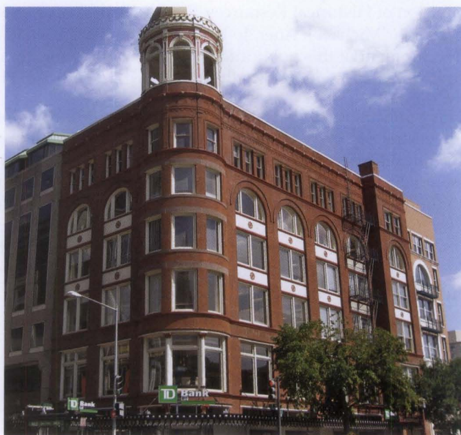
Figure 30. The small addition on the right of this late-19th century commercial structure is clearly secondary and compatible in size, materials and design with the historic building.
