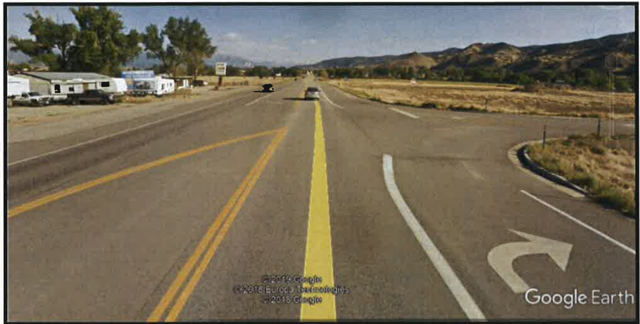
Figure 8-Highway 50 looking North West at Vandaveer Ranch Road
