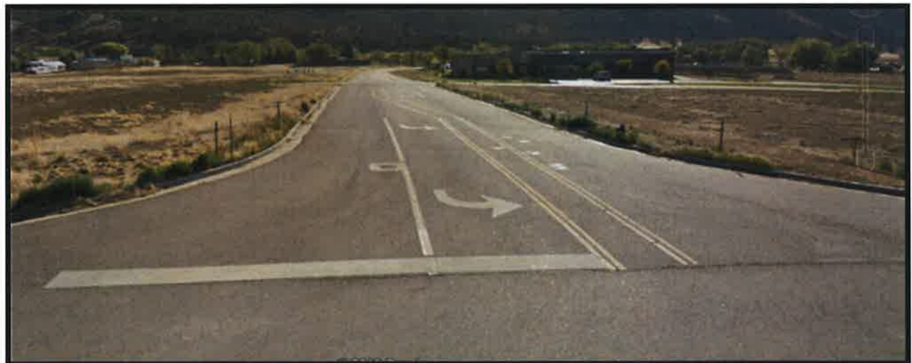
Figure 9-Vandaveer Ranch Road looking East from Highway 50
