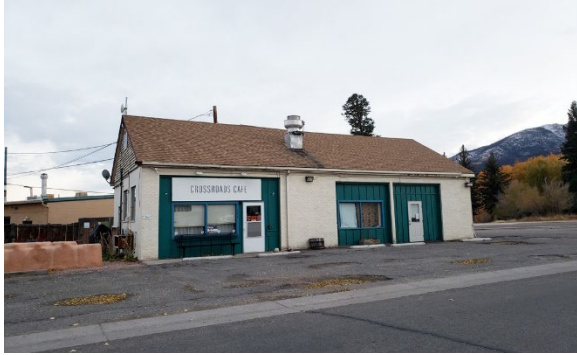
Photo 53: Former service station, 142 West US 50.
