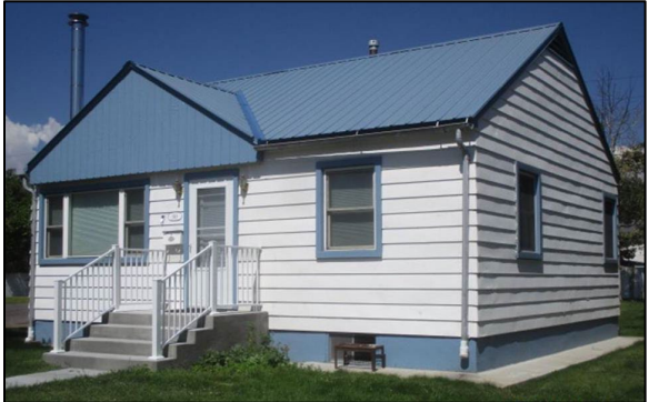
Photo 63: Minimal Traditional type house at 948 G Street (Source: Chaffee County Assessor)
