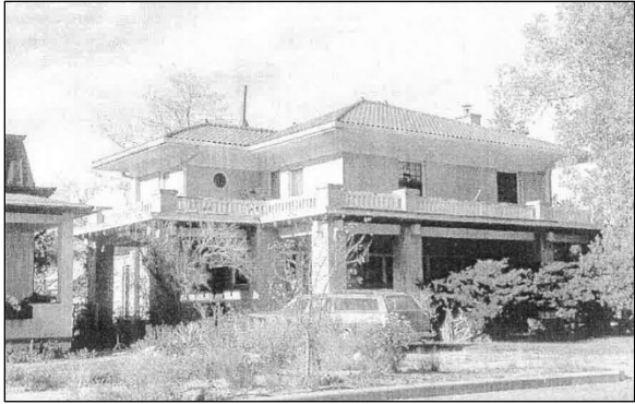
Photo 18: Cochems House, 408 F Street (5CF.2042) found potentially Eligible to the NRHP.
