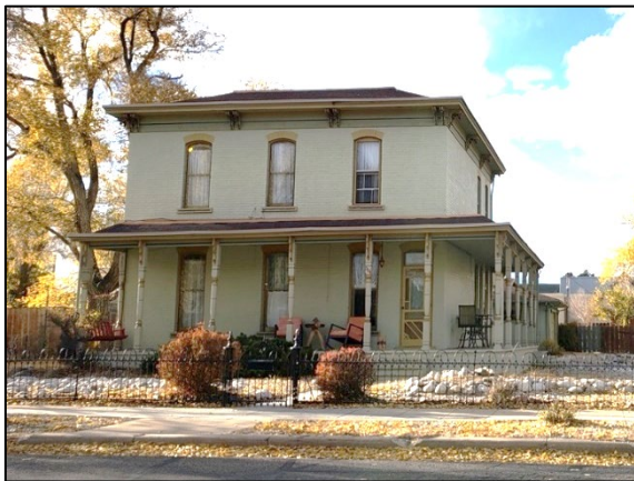
Photo 60: Italianate Style residence, 506 G Street.
