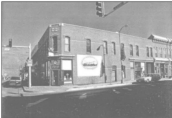
Photo 14: Twitchell Building, 101 N. F Street (5CF.406.45).
