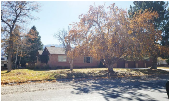
Photo 55: Post-WWII Ranch type residence, 525 Poncha Boulevard, built 1952.
