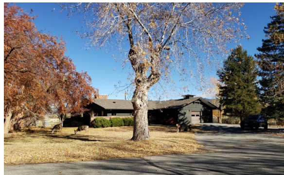
Photo 49: A later Eddy Brothers Addition Ranch type residence built in 1967, 500 Ouray Avenue.
