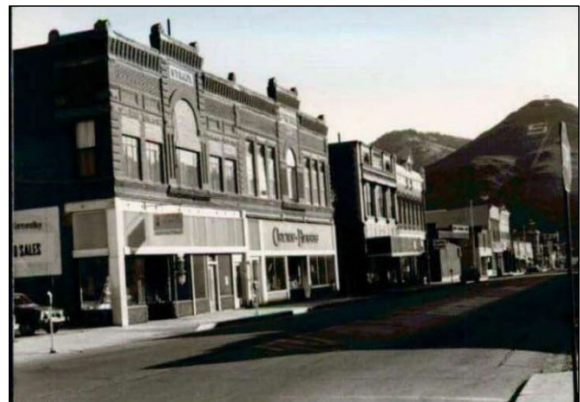
Photo 9: McKenna Building, 230 F Street (5CF.406.18).
