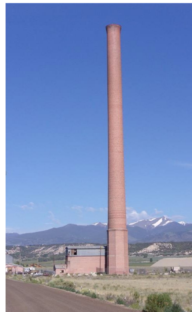
Photo 50: Ohio and Colorado Smelting Company Smokestack.
