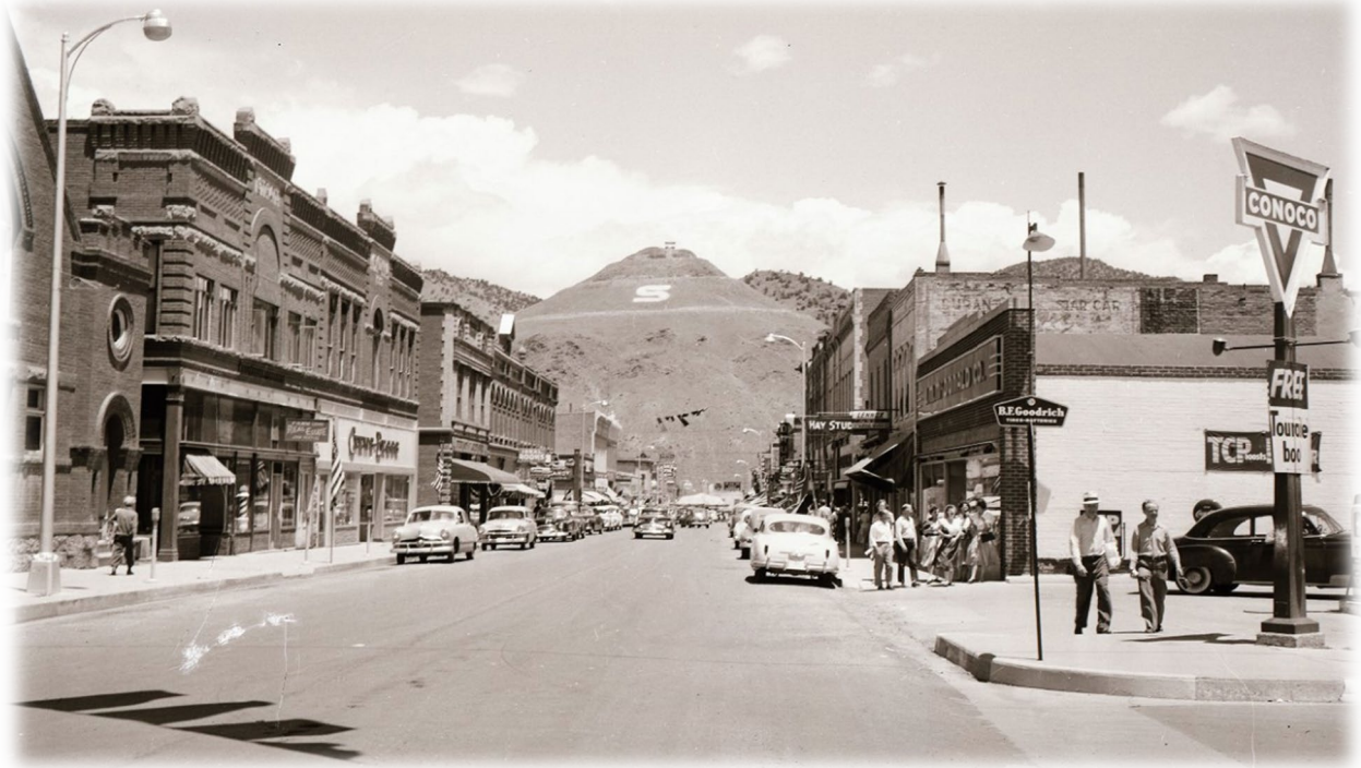
Photo 1. Downtown Salida, ca.1950 (photo courtesy of Salida Regional Library, Salida, Colorado)
