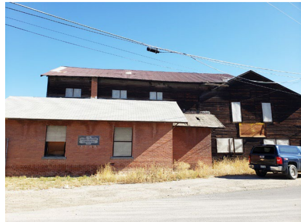
Photo 52: Former Salida Granite Company built in 1903, 348 H Street.
