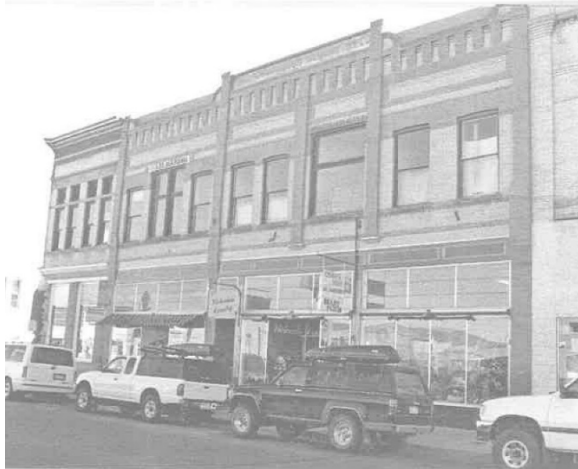
Photo 72: 207 F Street (2001 Downtown Survey)
