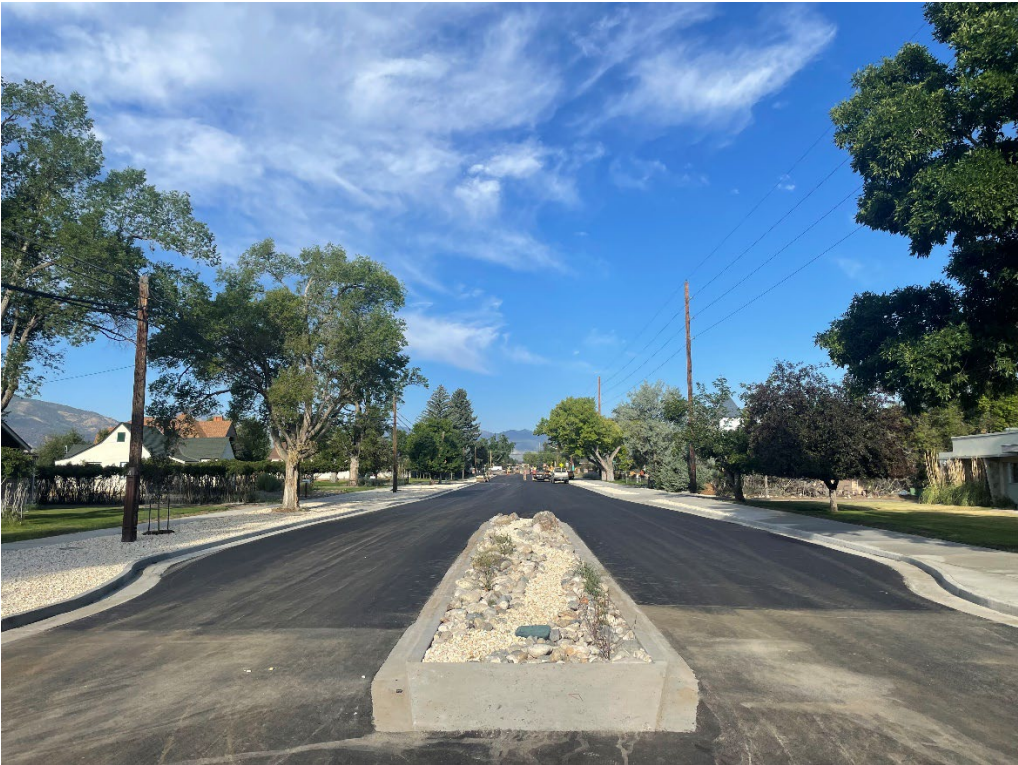
Figure 1 - Poncha Blvd Paving and Island at 5th
