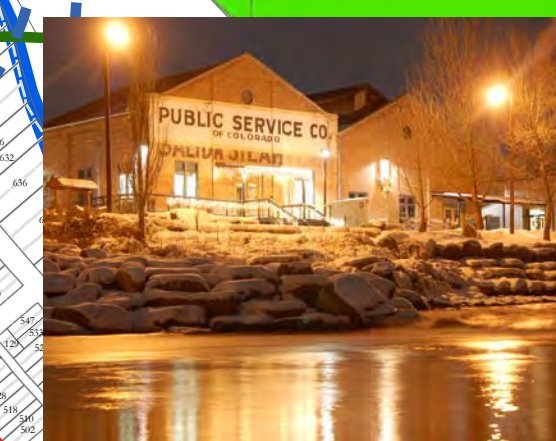
Salida Steam Plant
