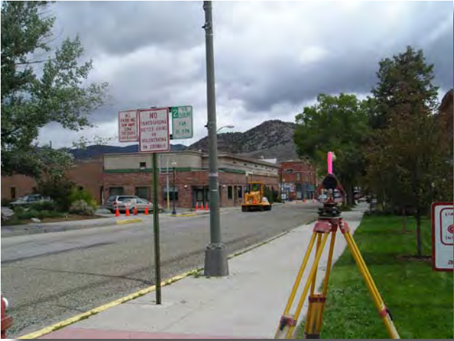
Chip seal project F Street
