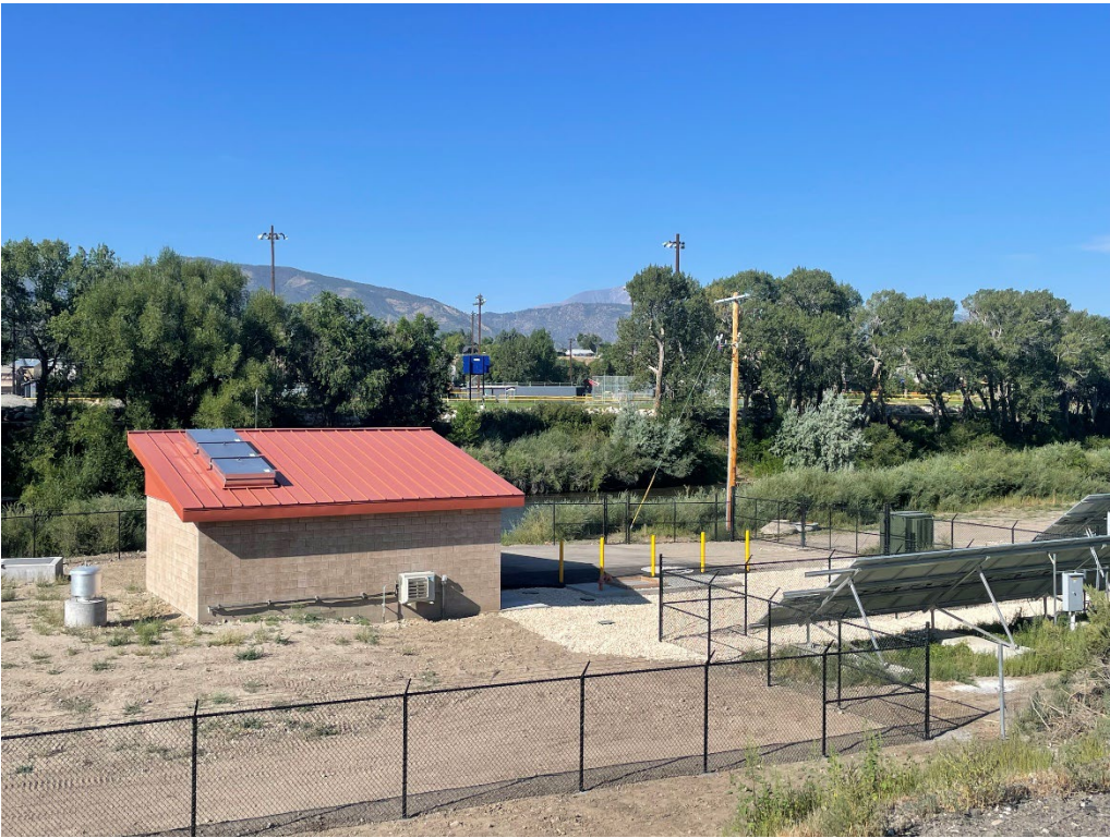
Figure 2 - Pump Station Building
