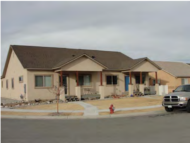
New Habitat for Humanity duplex at Starbuck Circle
