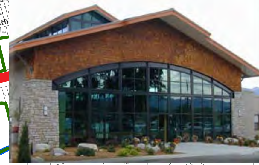
Salida Hot Springs Aquatic Center
