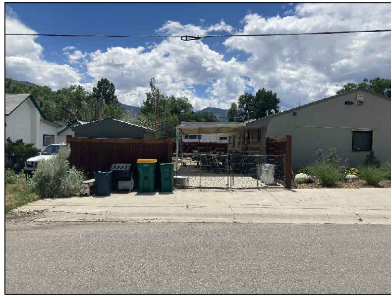
SOUTHEAST SIDE - 13TH STREET COVERED PORCH AREA
