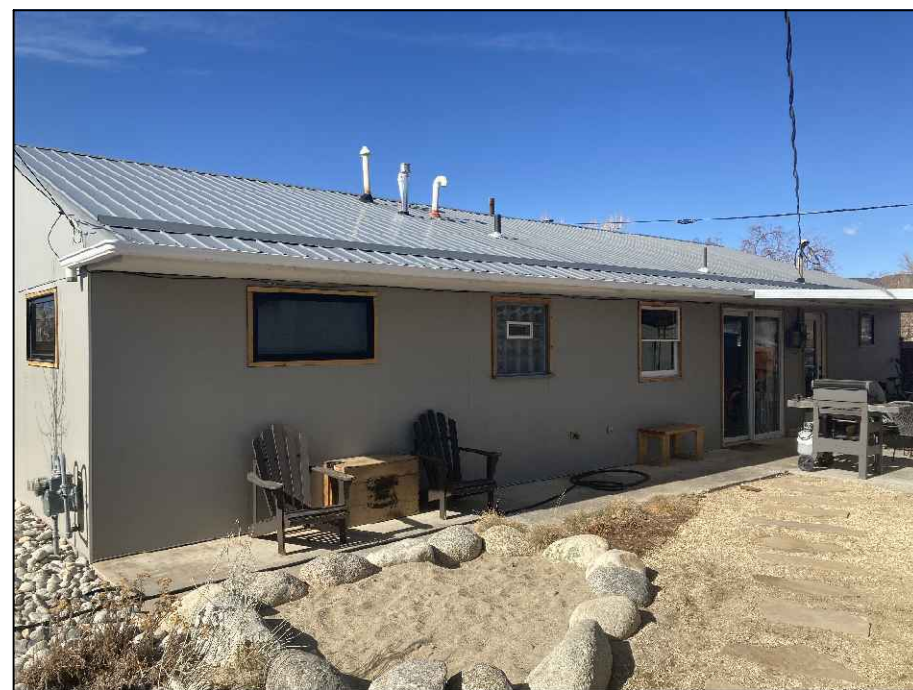
SOUTHWEST SIDE - REAR
