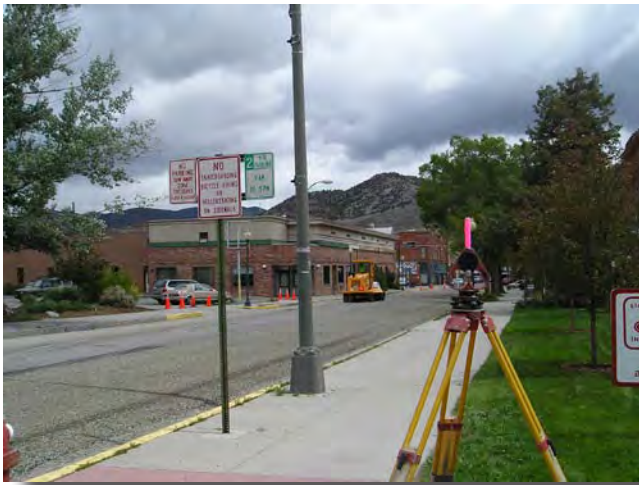
Chip seal project F Street
