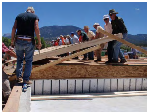
Wall raising at Starbuck Dairy Subdivision duplex Habitat for Humanity
