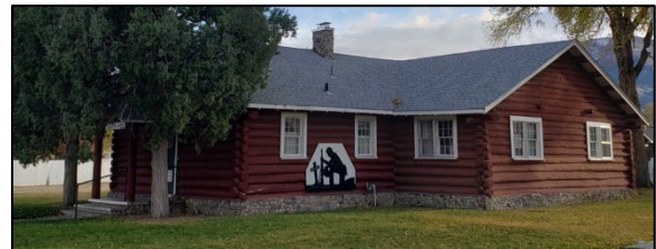
Photo 54: Rustic style American Legion Building at 235 W. 10 th Street
