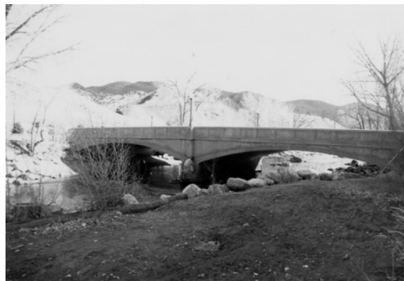
Photo 33: F Street Bridge over the Arkansas River (5CF.406.75)
