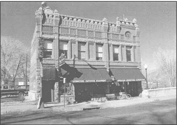
Photo 16: Bon Ton/Manhattan Hotel, 228 N. F Street (5CF.213)..
