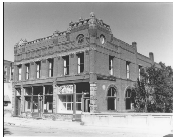
Photo 46: Manhattan Hotel (Source: NR Nomination)
