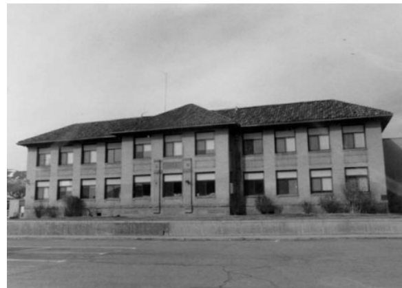
Photo 45: Kesner Memorial Building (5CF.1507)
