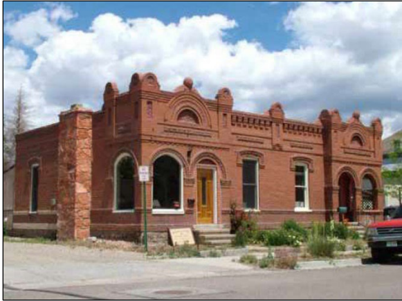
Photo 24: Parlin Terrace, 120-122 C Street (5CF.2216) found potentially Eligible to the NRHP.
