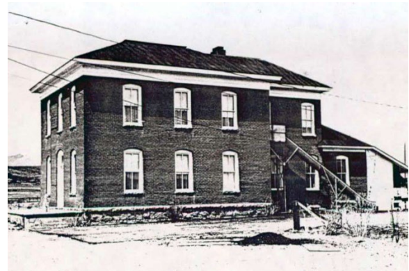
Photo 31: Chaffee County Poor Farm (5CF.190)
