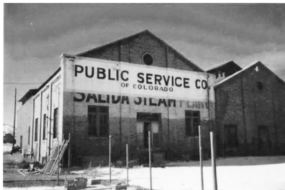
Photo 40: Edison Electric/Salida Steam Plant (5CF.291)
