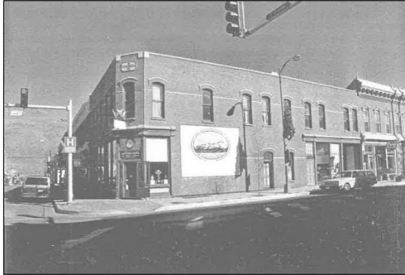
Photo 14: Twitchell Building, 101 N. F Street (5CF.406.45).
