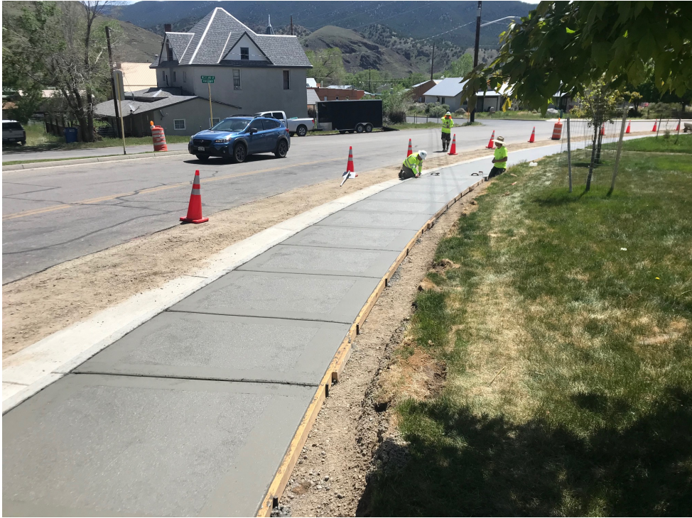
Figure 1 – Poncha Blvd and 3 rd St. Improvements
