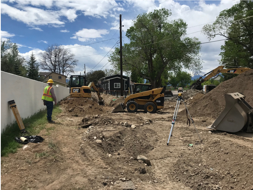
Figure 2 – Sewer Reconstruction near Pitkin and Ouray Ave.
