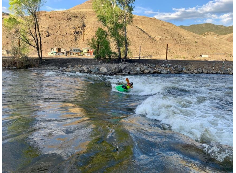
The Office Wave is an example of a drop structure.
