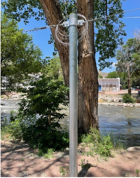
Steel slalom posts with longitudinal wires in Canon City.
