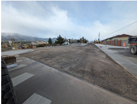
Poncha Blvd and Holman Reconstruction
