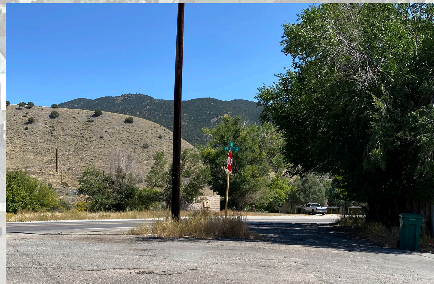
4 The intersection of CO 291 and Walnut St. will be rebuilt to replace existing open asphalt with curb and gutter, curb returns, and pedestrian facilities.
