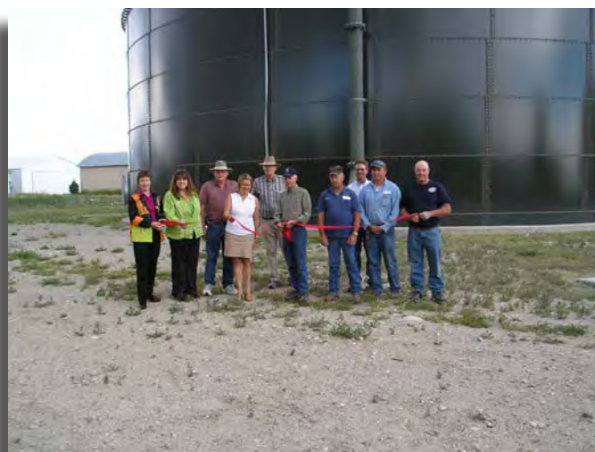
New water tank at the airport
