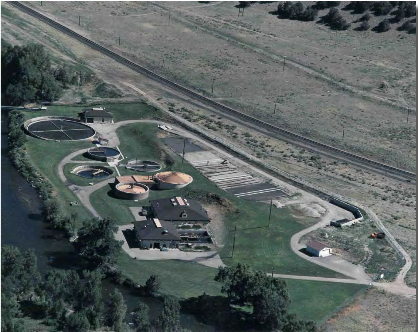
Wastewater Treatment Plant built in 1956 renovated in 1985
