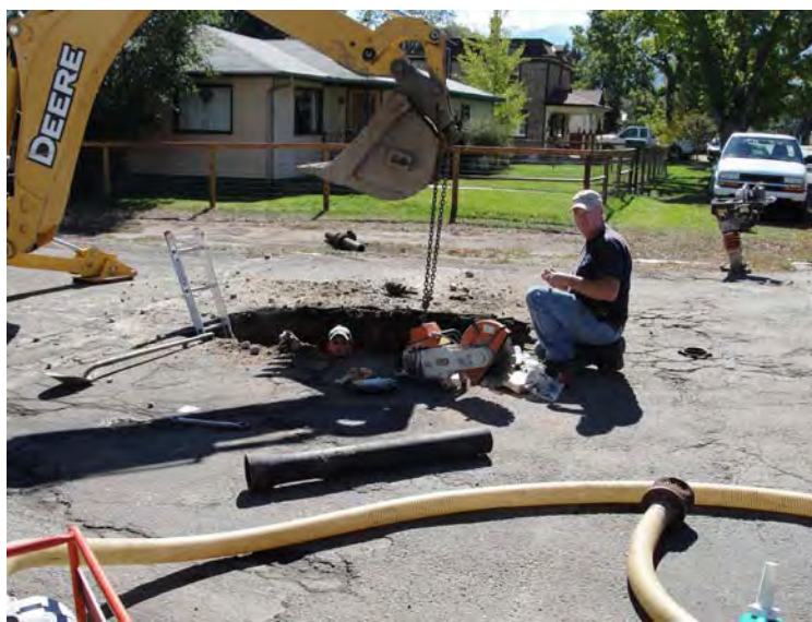
Public Works Repairing Water Lines
