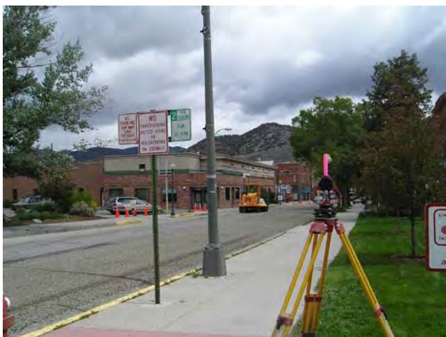
Chip seal project F Street
