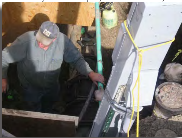
Public Works performing maintenance of city water lines
