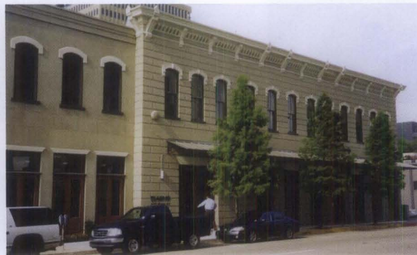
Figure 28. A small addition (left) was constructed when this 1880s train station was converted for office use. The paired doors with transoms and arched windows on the compatible addition reflect, but do not replicate, the historic building (right).
