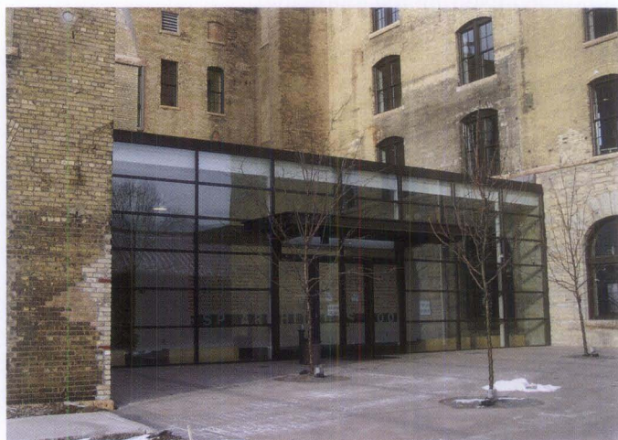
Figure 14. This glass addition was erected at the back of an 1895 former brewery during rehabilitation to provide another entrance. The addition is compatible with the plain character of this secondary elevation.
