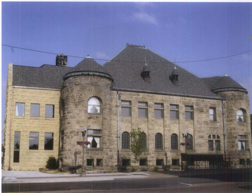
Figure 31. An elevator/stair tower was added at the back of this Richardsonian Romanesque-style theater when it was rehabilitated. Rough-cut stone and simple cut-out openings ensure that the addition is compatible and subordinate to the historic building. Photo: Chuck Liddy, AIA.
