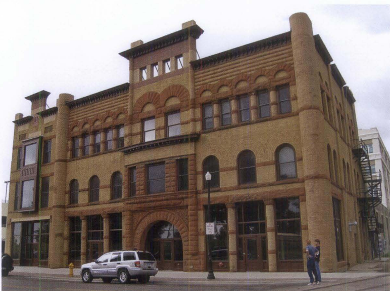
Figure 10. The small size and the use of matching materials ensures that the new addition on the left is compatible with the historic Romanesque Revival-style building.
