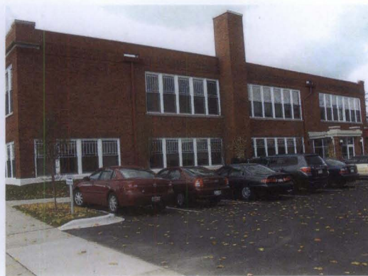
Figure 29. This simple glass and brick entrance (left) added to a secondary elevation of a 1920s school building (right) is compatible with the original structure.
