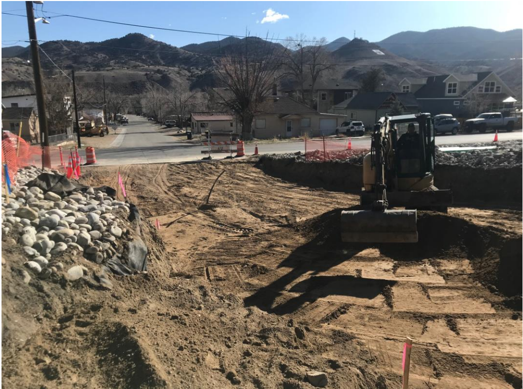
Figure 2 - E. Crestone Road Construction
