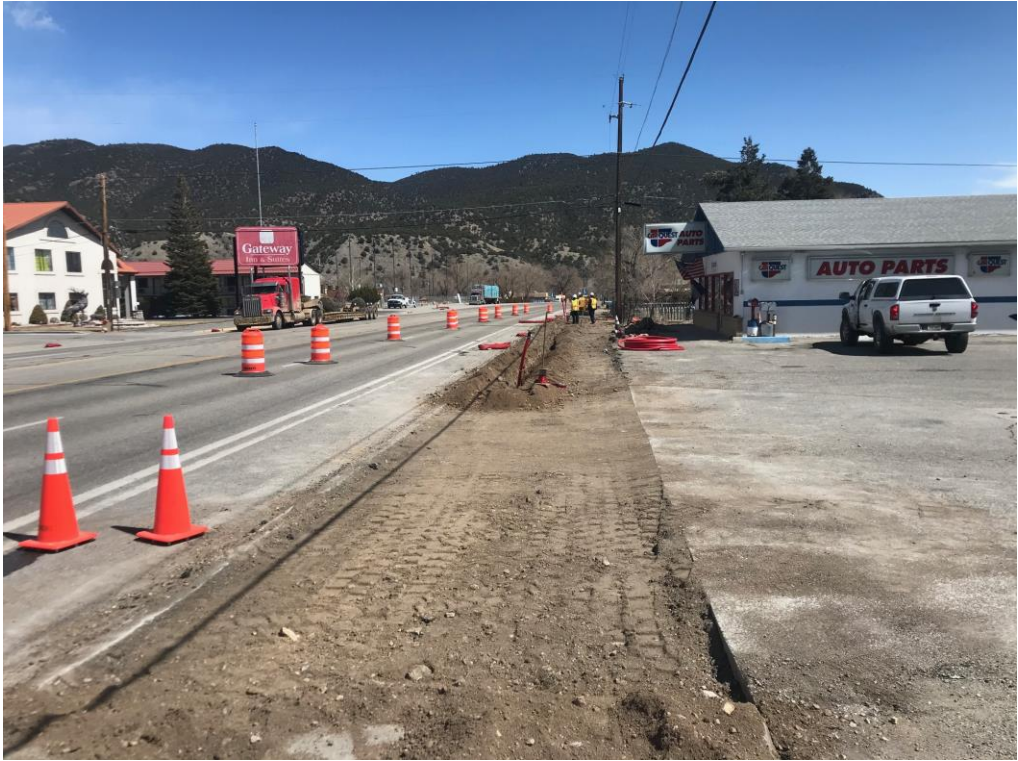
Figure 1 - US-50 Phase IV Streetscape Construction
